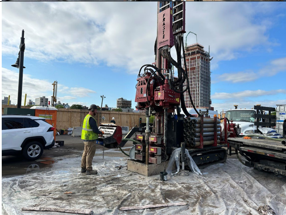
Photo 2: View of Coastal Environmental Solutions drilling DB-2 with Sonic Drill Rig CRS XL 140 DUO
