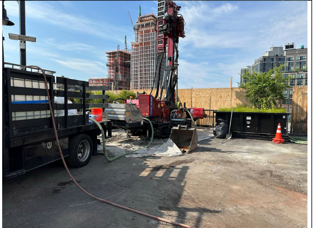
Photo 2: View of Coastal Environmental Solutions drilling DB-4 with Sonic Drill Rig CRS XL 140 DUO
