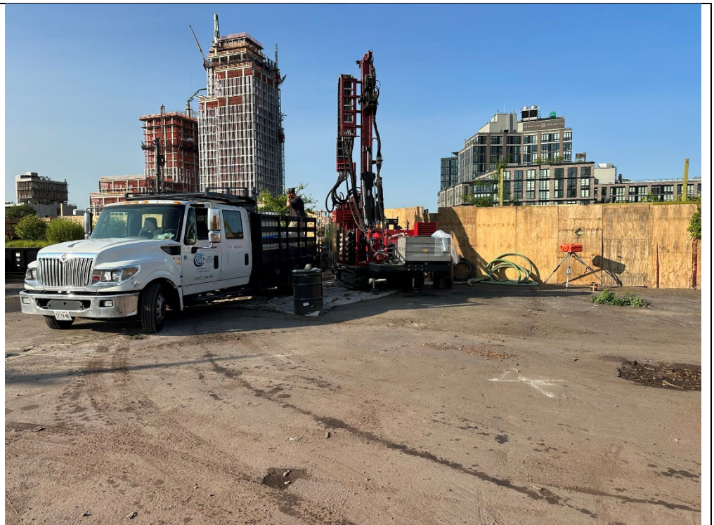
Photo 1: View of CAMP station and Coastal Environmental Solutions drilling DB-6 with Sonic Drill Rig CRS XL 140 DUO
