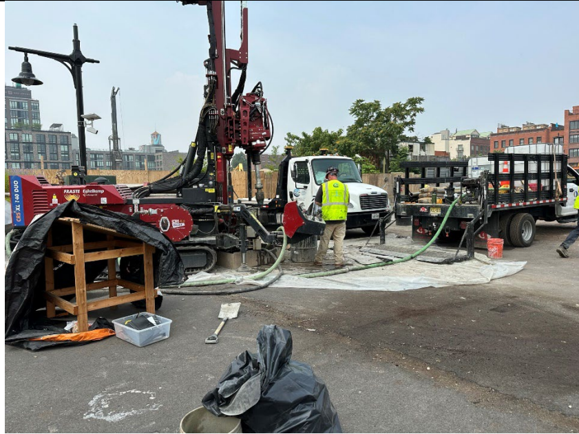
Photo 3: View of grouting at DB-5.
