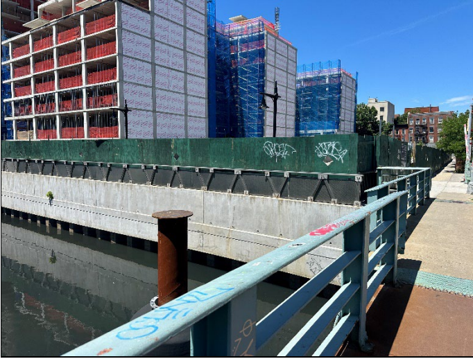
1. View of high-level relieving platform and sheeting, facing southwest.
