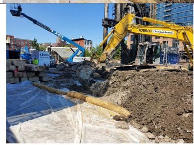
Photo 4: View of remaining spoils covered with poly sheeting, facing south.
