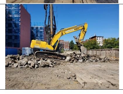
Photo 4: View of GSI chopping concrete debris with the hammer attachment, facing northwest.
