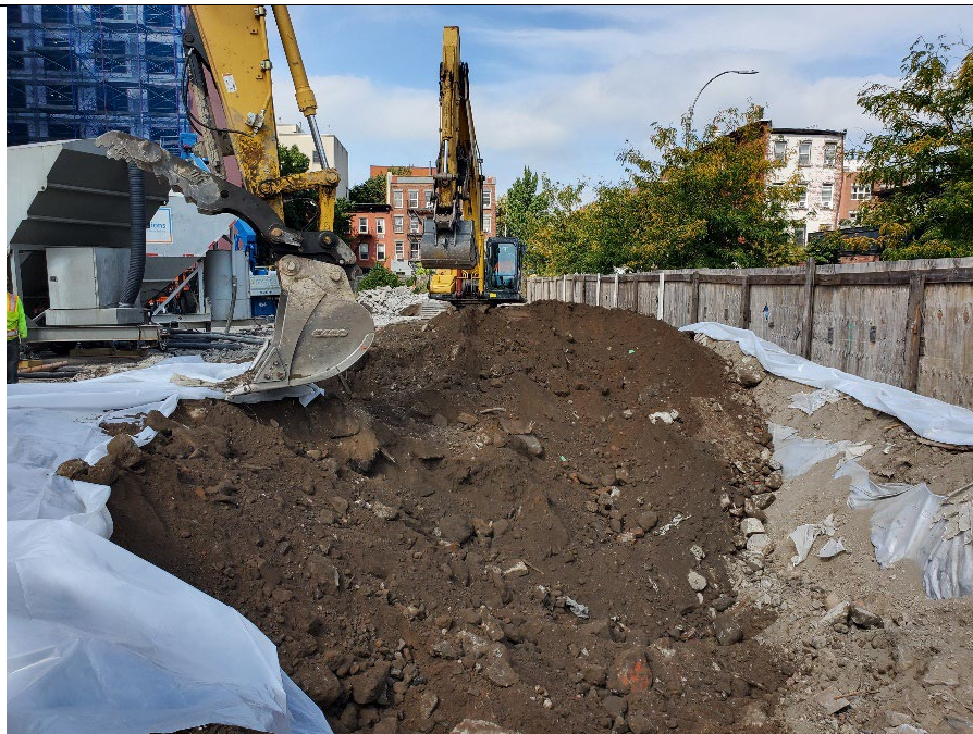
Photo 3: GSI excavating for berm installation, facing west.
