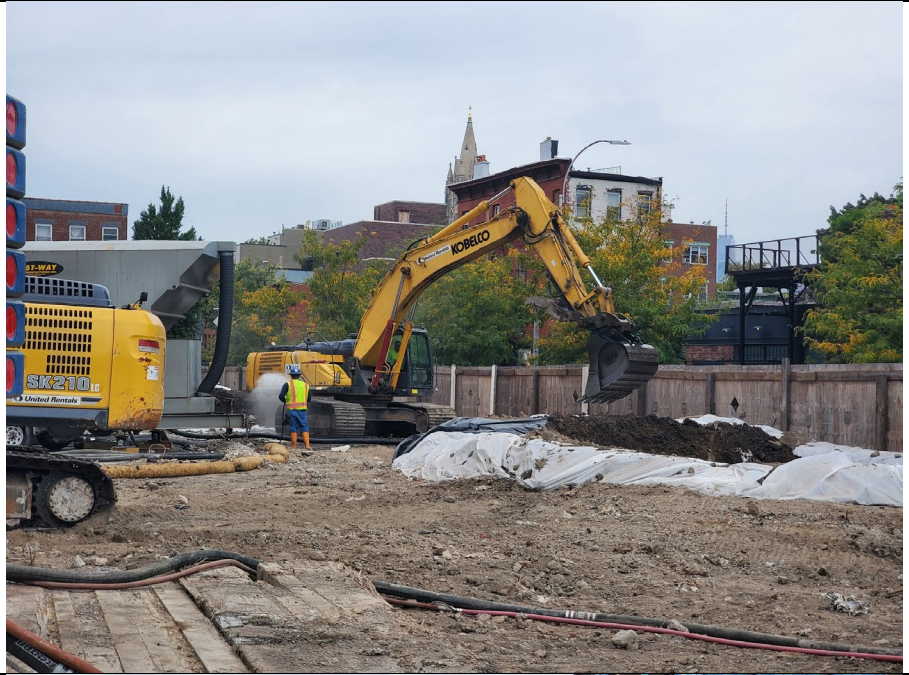
Photo 3: GSI moving spoils staged within the berm onto poly-sheeting on the western portion of the site, facing northwest.
