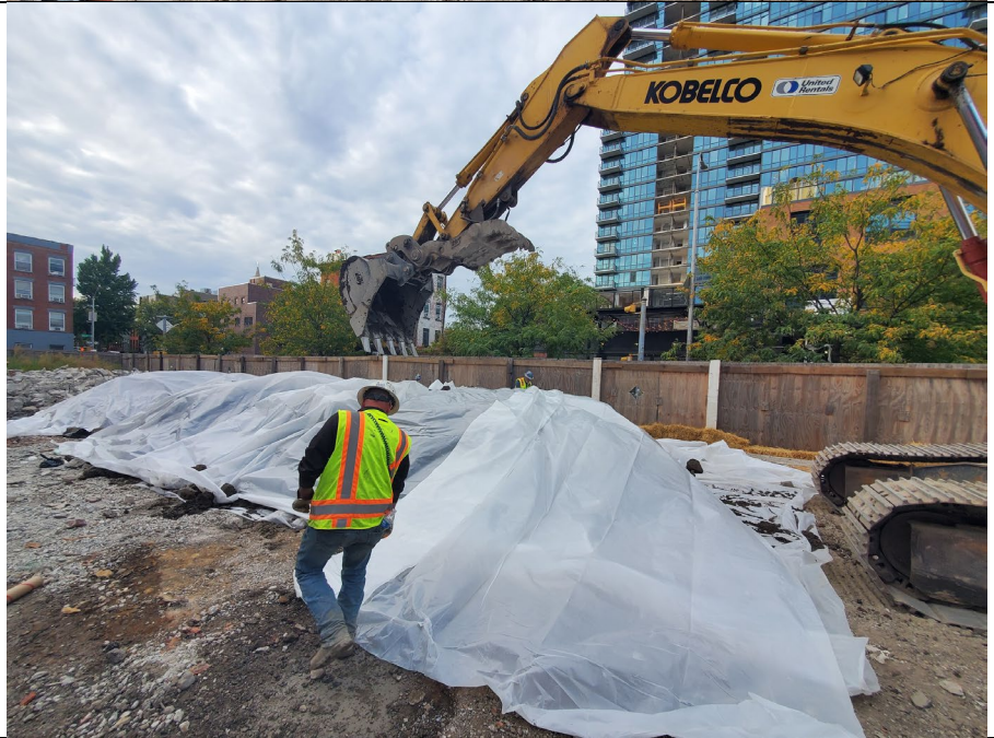
Photo 4: GSI covering spoil stockpile with poly-sheeting, facing northwest.
