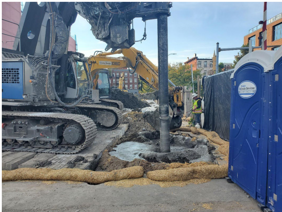
Photo 3: View of GSI introducing 9% mixture at column/cell E11, facing west.
