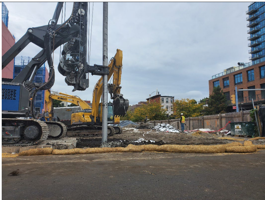
Photo 3: View of GSI introducing 9% mixture at column/cell C7 with application of foam to mitigate odors, facing west.
