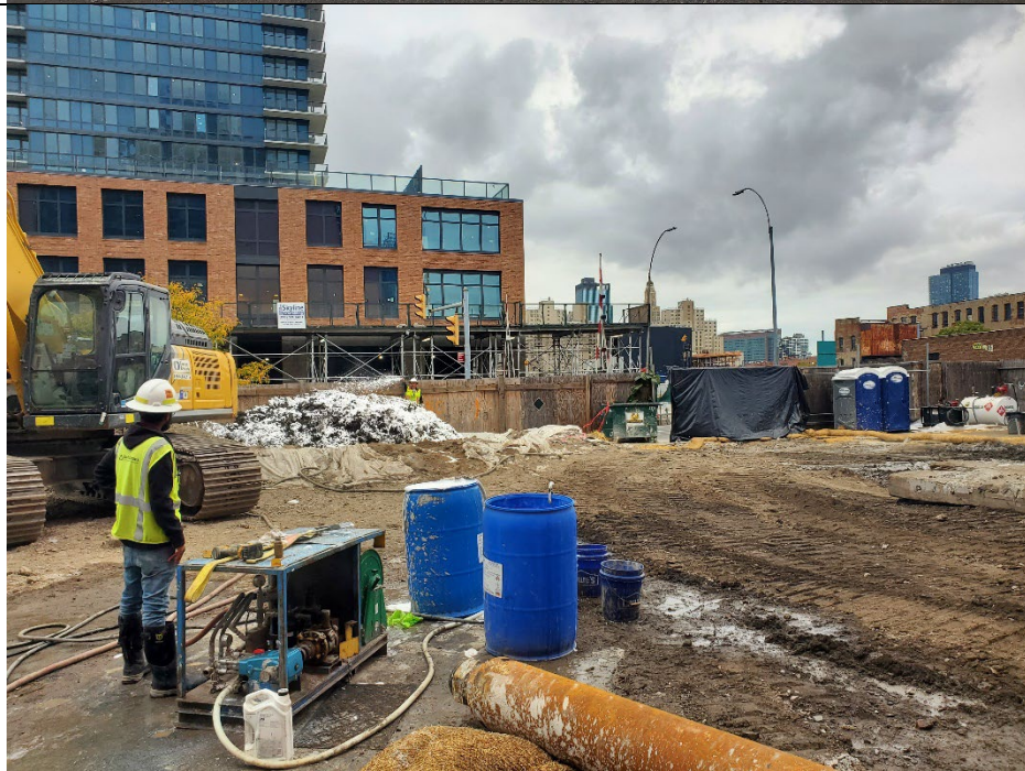
Photo 4: GSI applying foam on top of spoils within berm, facing north.
