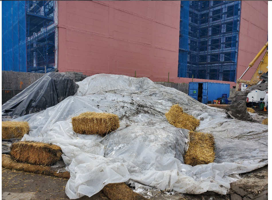
Photo 4: Poly sheeting is placed atop of ISS spoils and secured at the end of the day, facing southwest.
