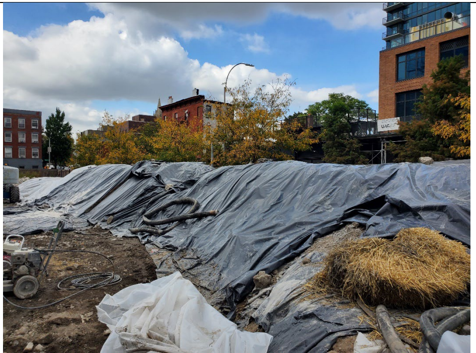
Photo 5: Poly sheeting is placed on top of ISS stockpile and secured at the end of the day, facing northwest.
