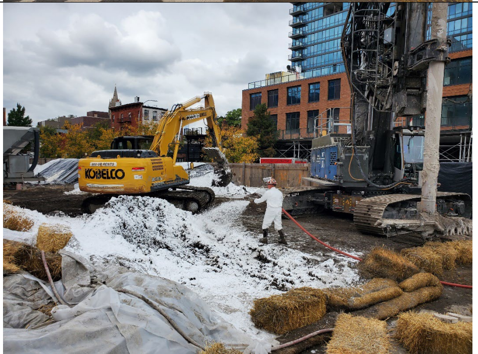
Photo 2: GSI applying foam restaging of ISS- spoils into the berm, facing northwest.
