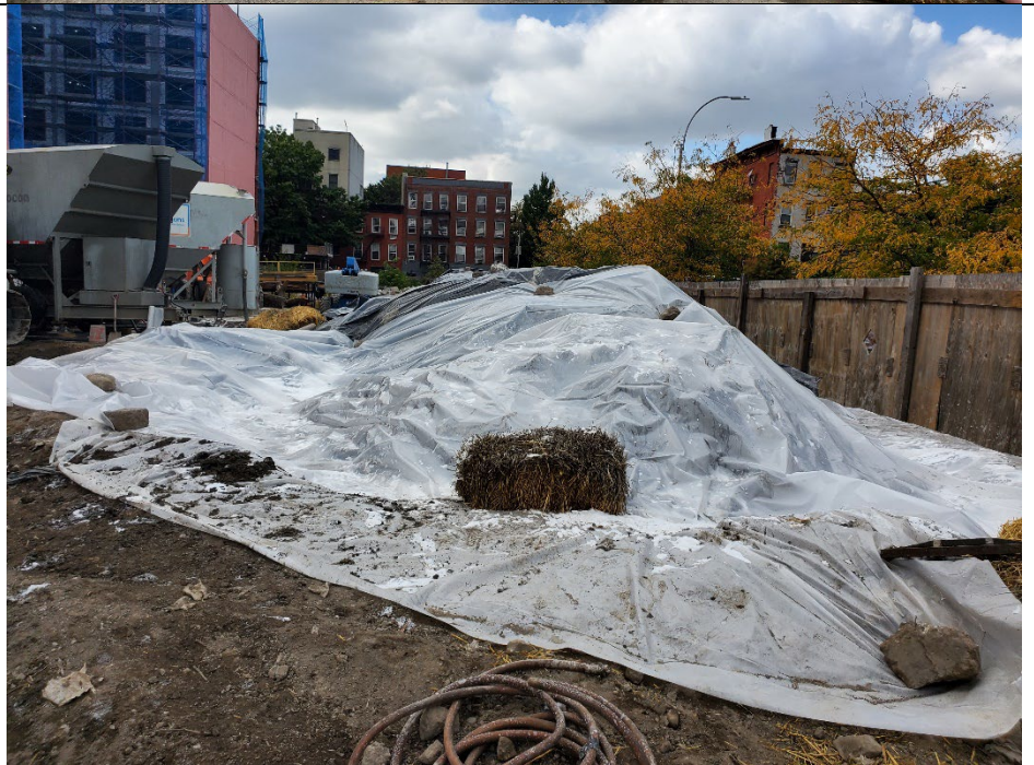
Photo 4: Poly sheeting is placed atop of ISS spoils within the berm and secured at the end of the day, facing west.
