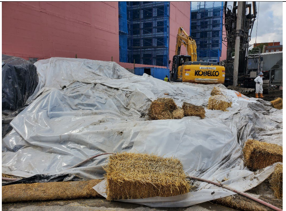
Photo 3: Poly sheeting is placed atop of ISS spoils and secured at the end of the day, facing southwest.
