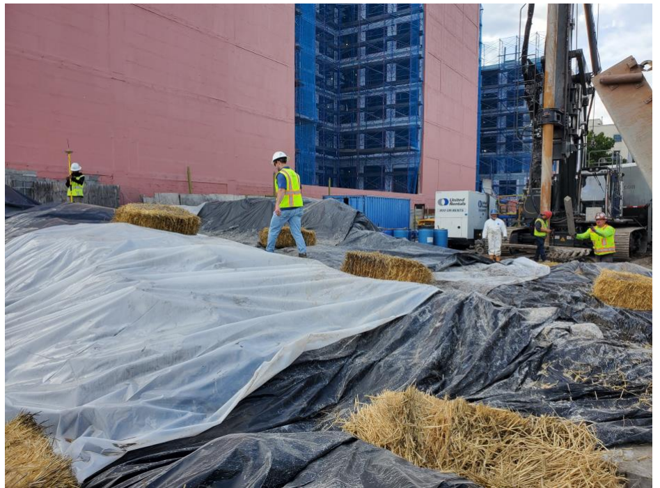
Photo 4: Poly sheeting placed atop ISS spoils and secured after reshaping, facing southwest.
