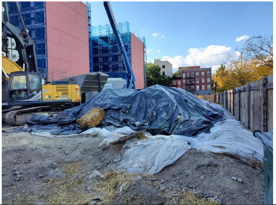
Photo 5: Poly sheeting placed on top of berm with ISS material and secured at the end of the day, facing west.
