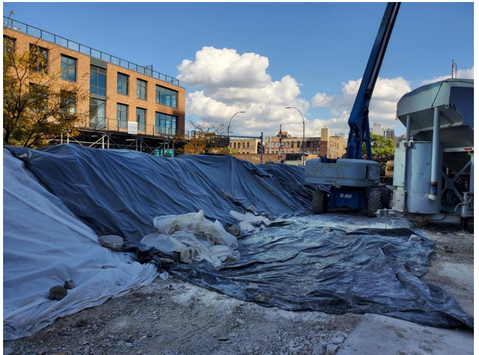
Photo 6: Poly sheeting on top of the north stockpile secured at the end of the day, facing west.
