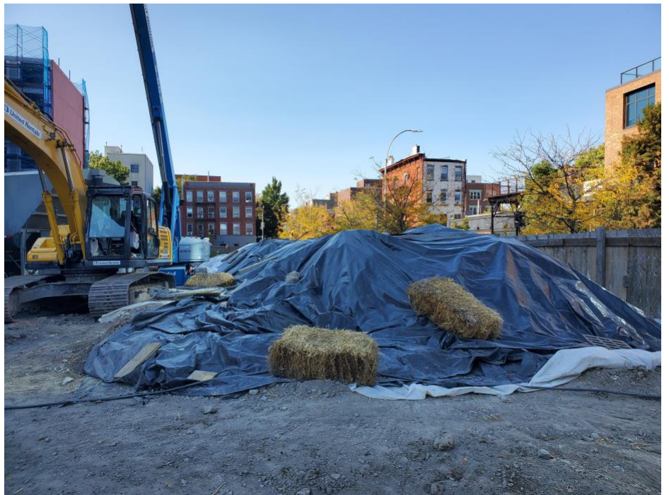
Photo 6: Poly sheeting placed atop of ISS spoils within the berm and secured at the end of the day, facing west.
