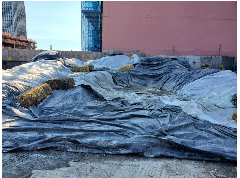
Photo 5: Poly sheeting placed atop of ISS spoils and secured at the end of the day, facing south.
