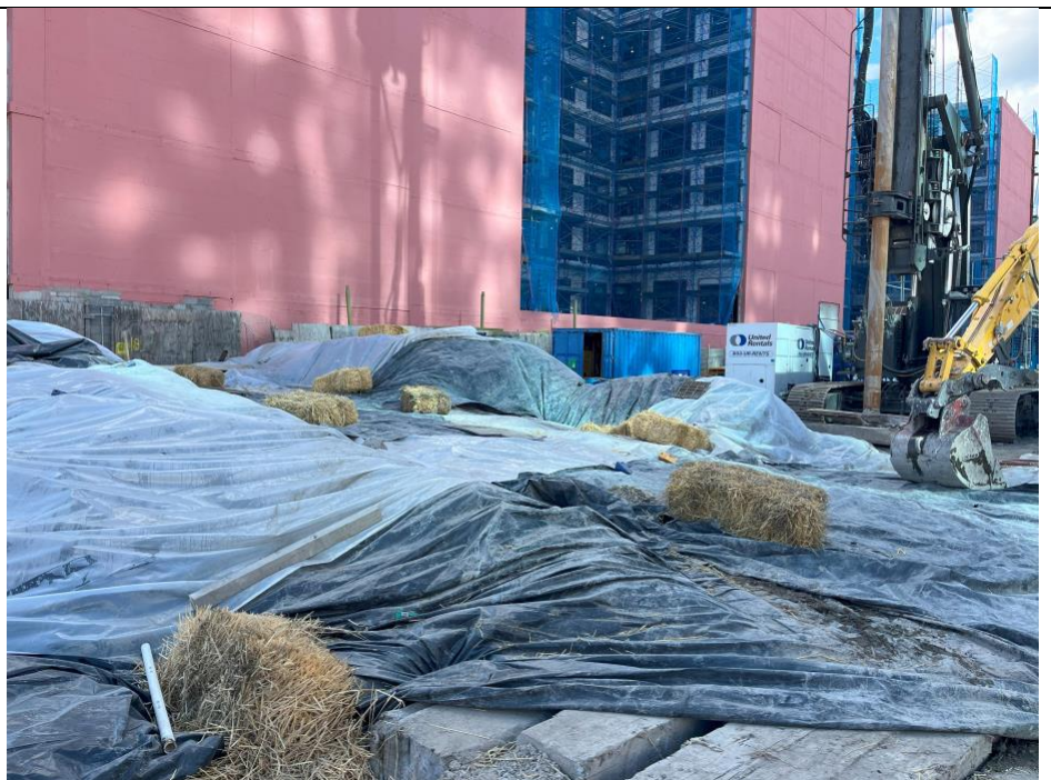
Photo 6: Poly sheeting placed atop of ISS spoils and secured at the end of the day, facing south.
