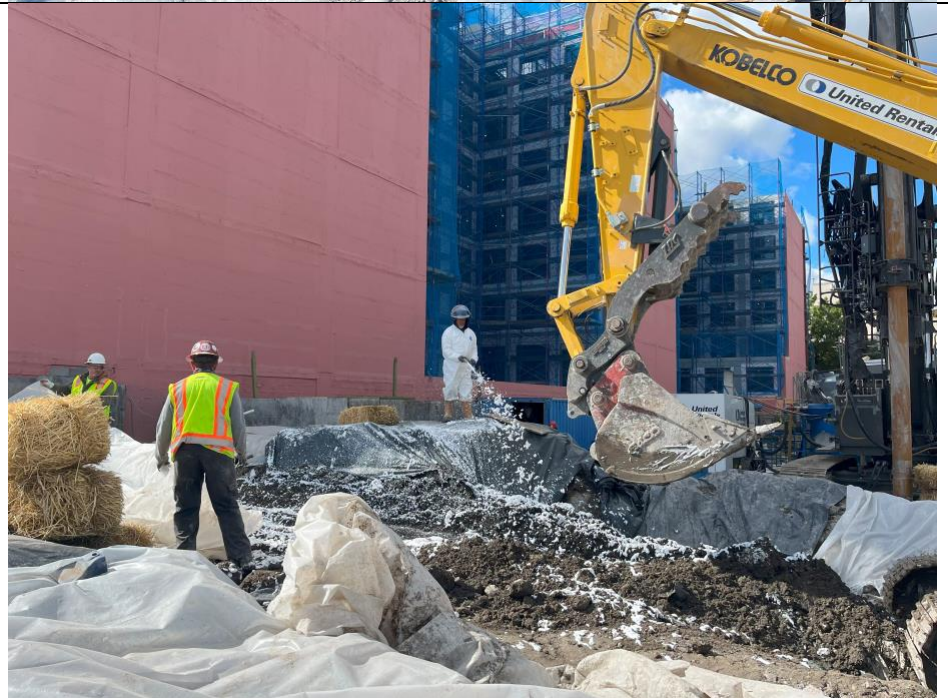
Photo 2: Moving and grading stockpile while applying foam deodorizer
