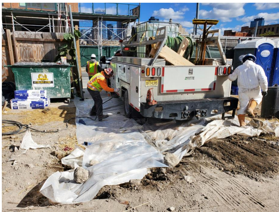
Photo 4: GSI cleaning the tracks for the Craig's truck on top of poly sheeting, view facing north.
