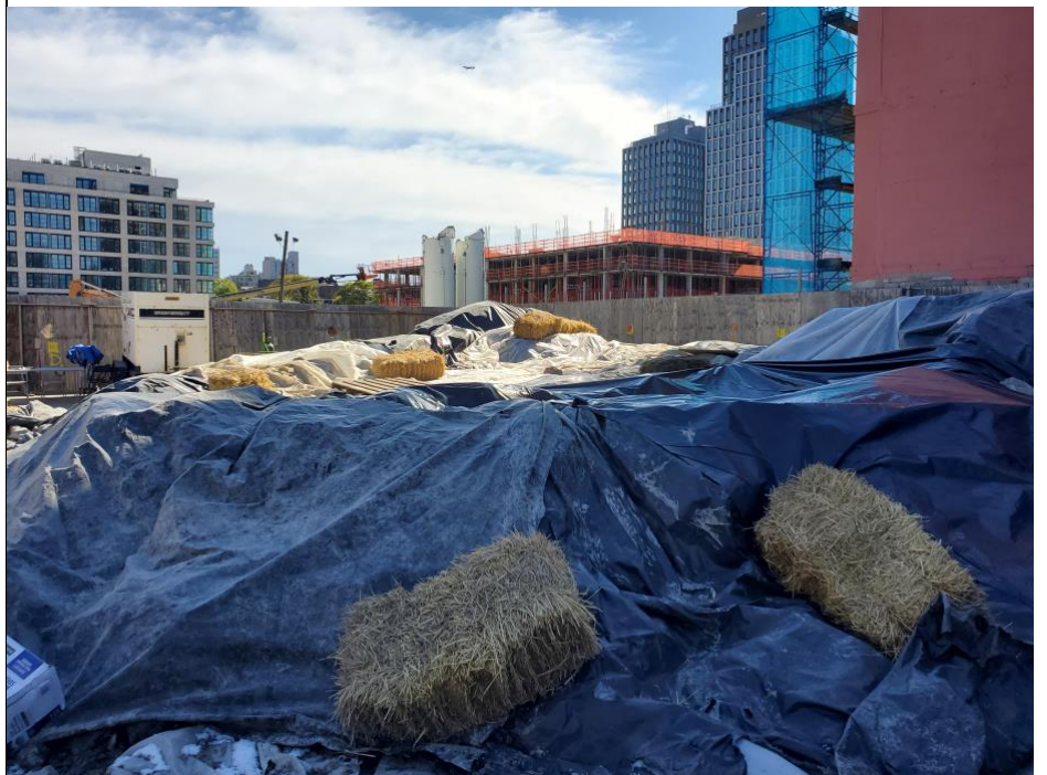
Photo 4: Poly sheeting placed atop of ISS spoils and secured at the end of the day, facing southeast.
