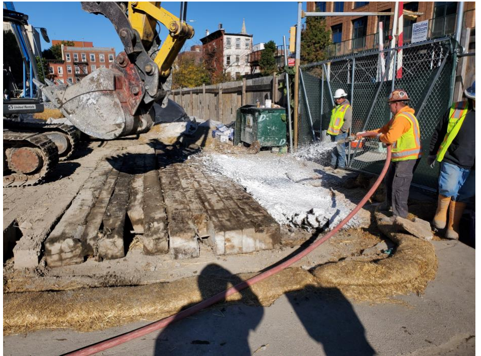
Photo 2: GSI applying foam while moving swell material, view facing northwest
