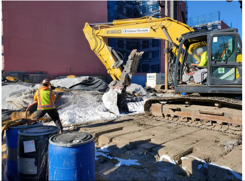
Photo 1: GSI applying foam while moving swell material, view facing southwest.
