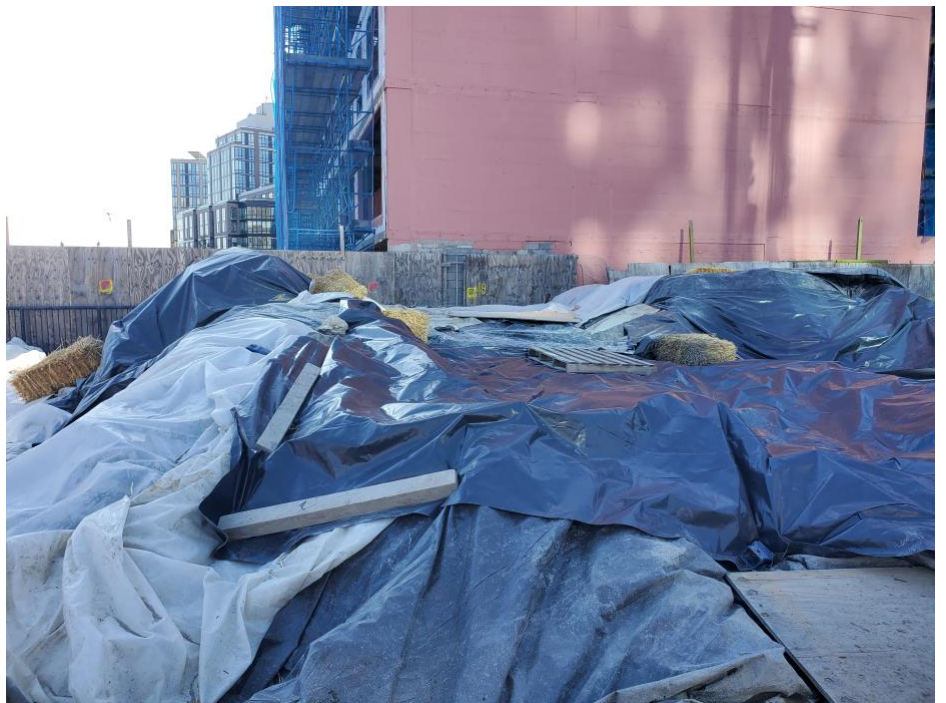
Photo 4: Poly sheeting placed atop of ISS spoils and secured at the end of the day, facing south.
