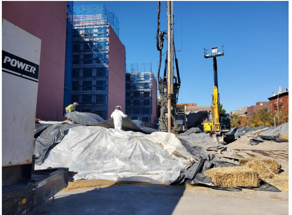
Photo 2: Poly sheeting replaced atop of ISS spoils and secured at the end of the day, facing west.
