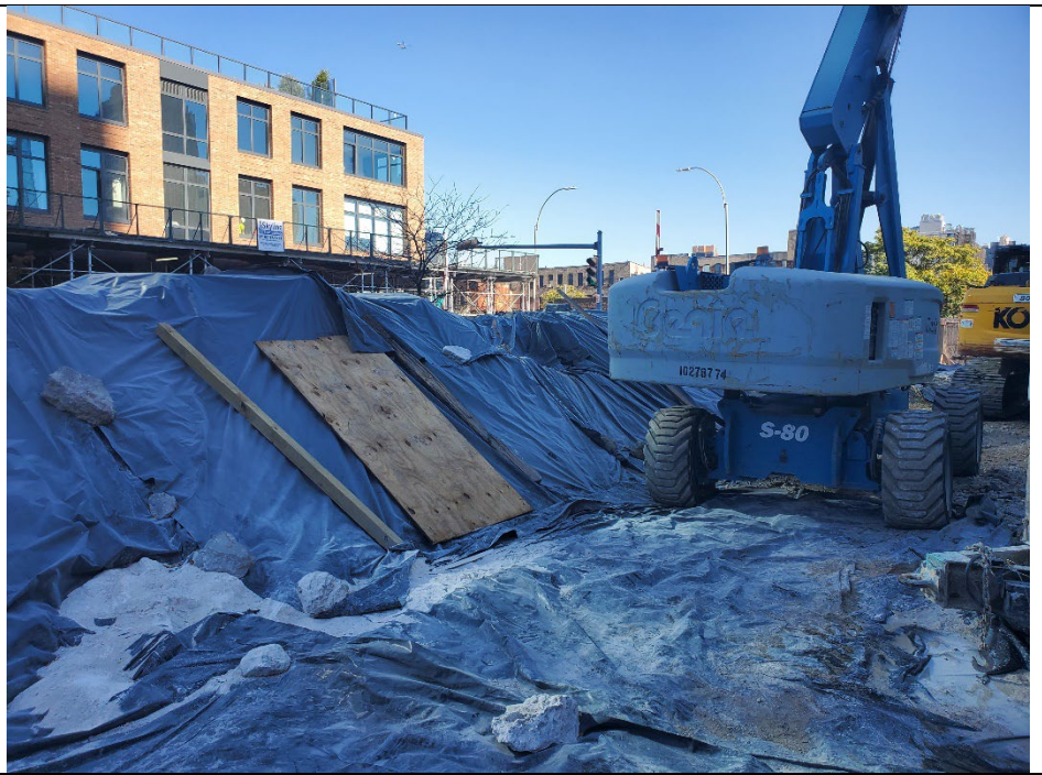
Photo 5: Poly sheeting placed on top of ISS spoils and secured at the end of the day, facing northeast.
