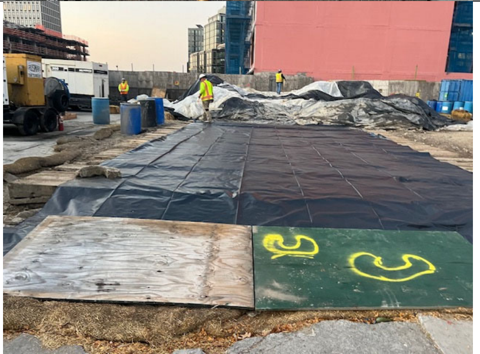
Photo 2: View of plastic sheeting placed on crane pad prior to the start of soil export, facing south.
