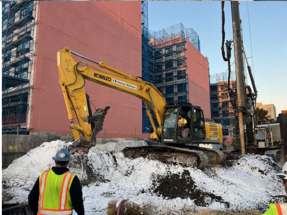
Photo 4: ISS spoils sprayed with odor suppression foam, facing southwest
