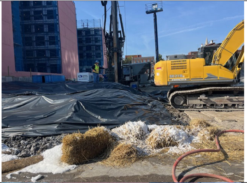
Photo 5: Poly sheeting placed atop of ISS spoils and secured at the end of the day, facing west
