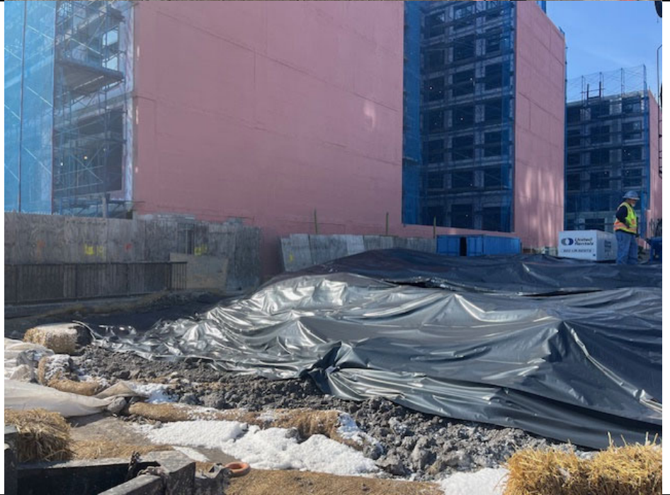
Photo 6: Poly sheeting placed atop of ISS spoils and secured at the end of the day, facing southwest
