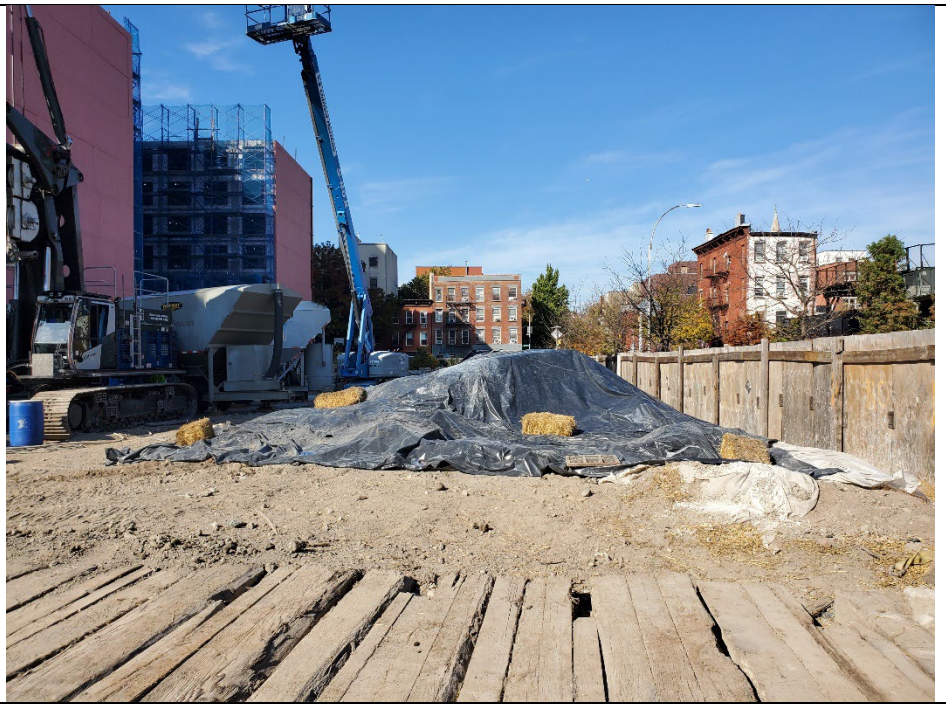
Photo 5: Poly sheeting placed atop of remaining ISS spoils and secured at the end of the day, facing west
