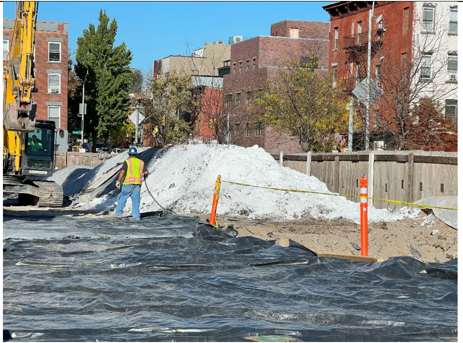
Photo 5: Exposed soil being foamed during the exportation of ISS Swell soil to Fairless Landfill in Morrisville, Pennsylvania, view facing northwest.
