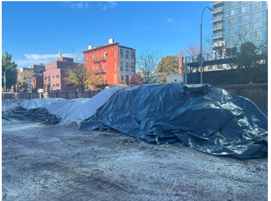
Photo 6: Poly sheeting placed atop of ISS spoils and secured at the end of the day, facing north.
