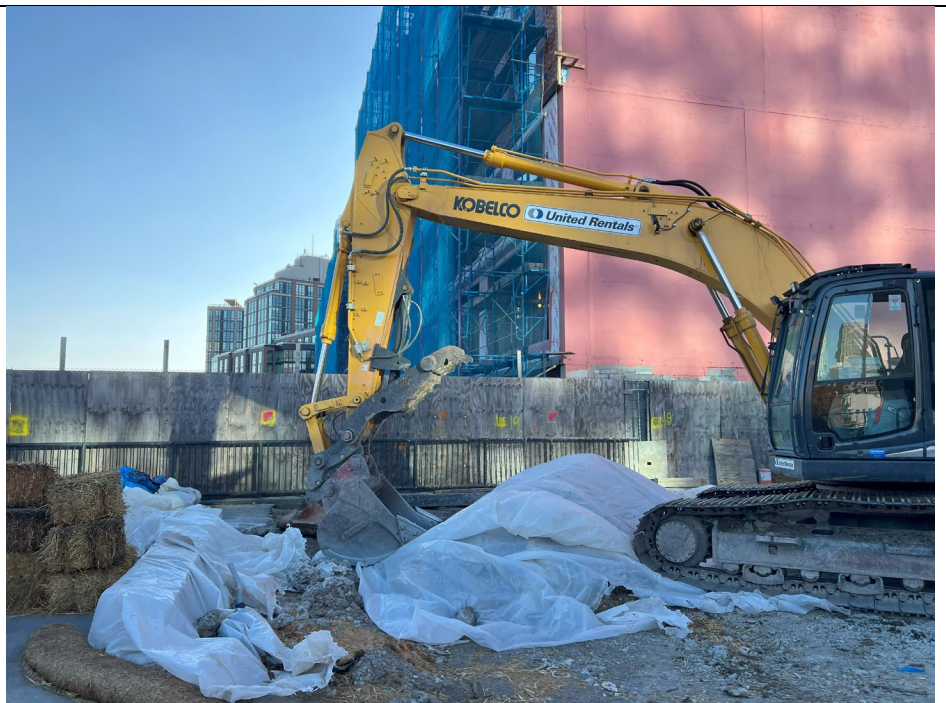
Photo 6: Poly sheeting placed swell soil and secured at the end of the day, facing south.
