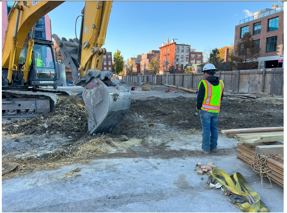
Photo 5: Removal of truck pad and regrading of soil, view facing northwest.
