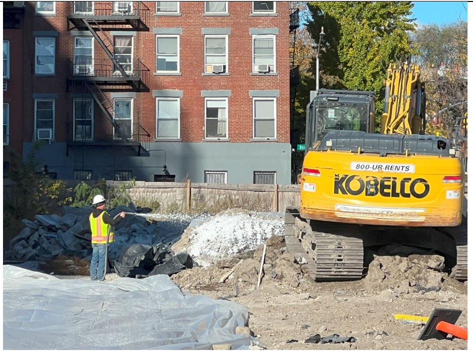
Photo 3: Exposed ISS swell material being foamed during exportation to Fairless Landfill, view facing west.
