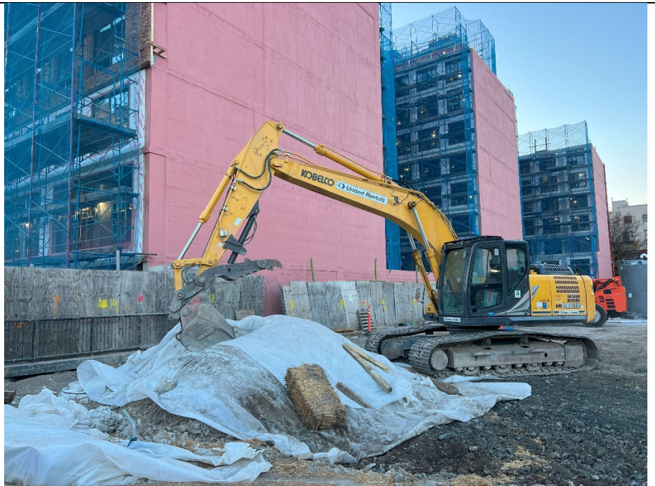
Photo 6: Poly sheeting placed on soil stockpile and secured at the end of the day, view facing south.
