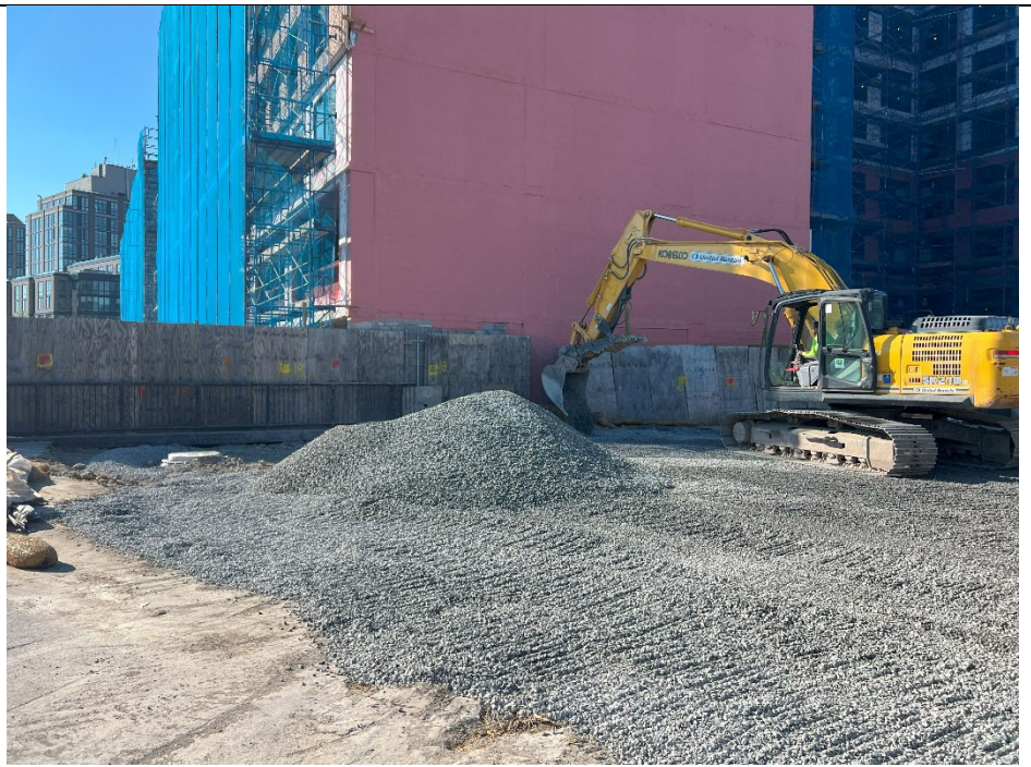
Photo 5: Grading of stone gravel backfill, view facing southeast.
