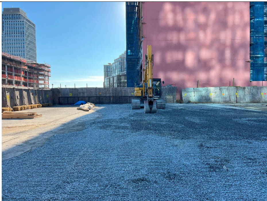
Photo 4: Graded stone gravel backfill, view facing south.
