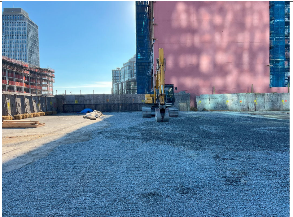
Photo 4: Graded stone gravel backfill, view facing south.
