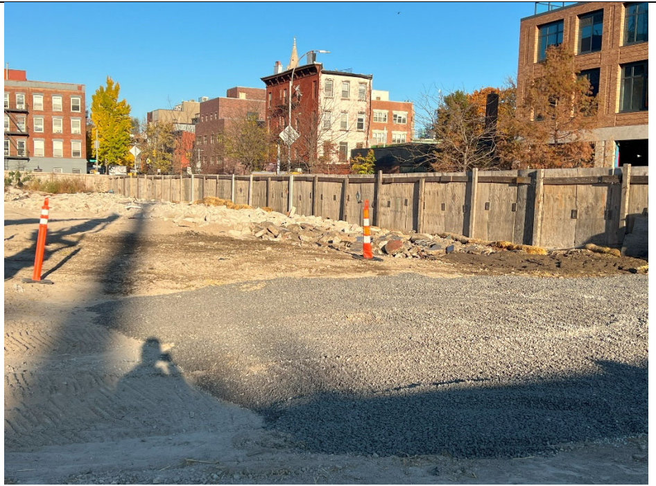
Photo 3: Grading of stone gravel backfill, view facing north.
