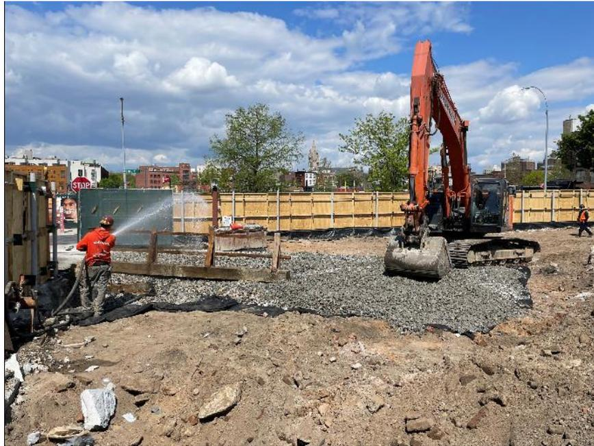
**Photo 1:** Mayrich spraying water to control dust and using ASTM #2 virgin stone to construct a stabilized construction entrance in the southwest portion of BCP Site No. C224309 (facing west)
