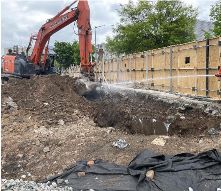
**Photo 1:** Mayrich excavating former foundation elements and spraying water to control dust in the southeastern portion of BCP Site No. C224309 (facing southeast)
