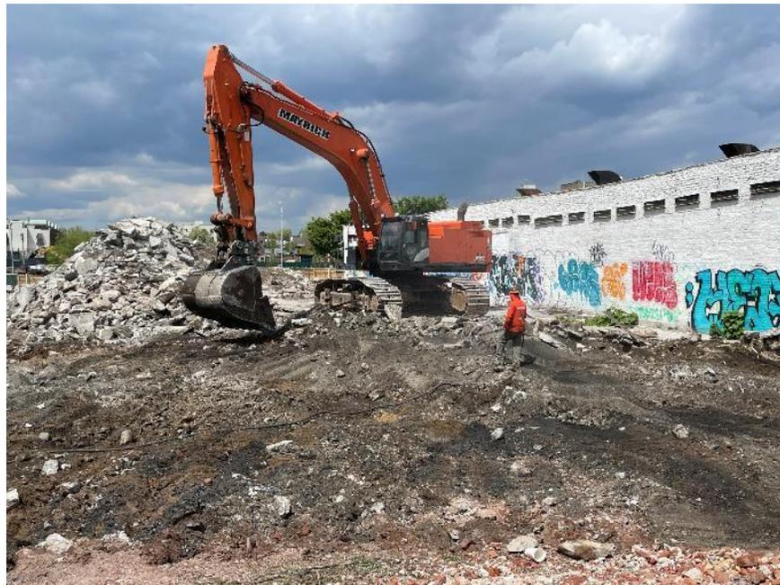
**Photo 2:** Mayrich stockpiling C&D debris in the northern portion of BCP Site No. C224220 (facing northwest)
