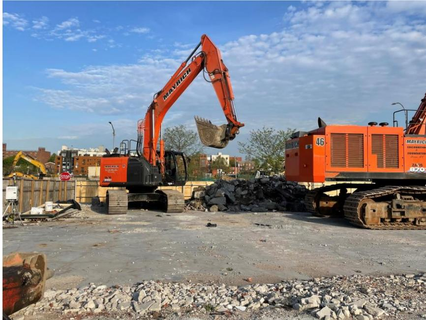
**Photo 1:** Mayrich stockpiling C&D debris in the northwestern portion of BCP Site NO. C224309 (facing west)
