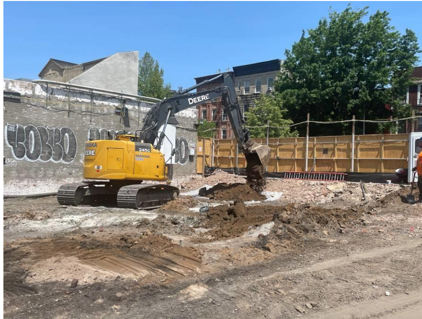
Photo 1: Skanska stockpiling spoils generated during pile advancement on polyethylene sheeting in the northeastern portion of BCP Site No. C224309 (facing northwest)
