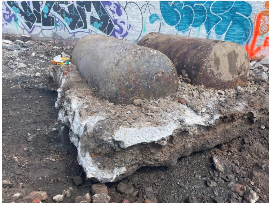
Photo 1: Two 550-gallon USTs partially encased in concrete uncovered in the northern portion of BCP Site No. C224220 (facing north)
