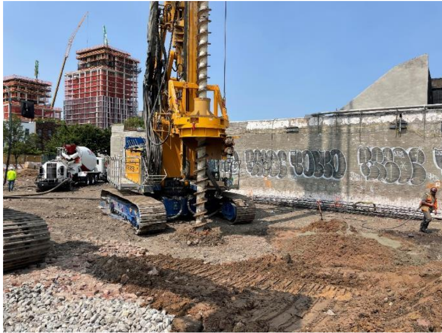
Photo 1: Skanska advancing auger for pile installation in the eastern portion of BCP Site No. C224309 (facing southwest)
