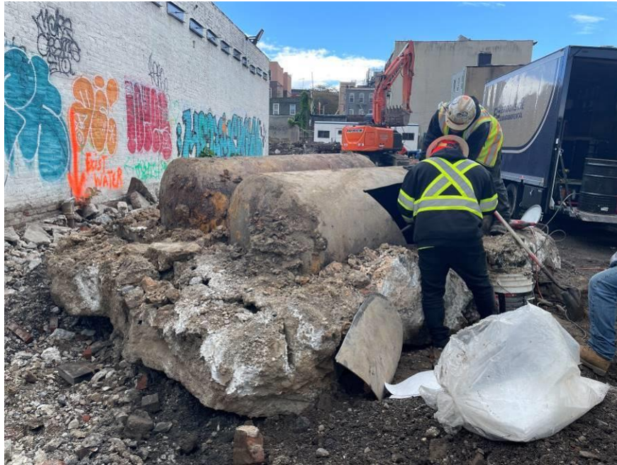
Photo 1: Brookside decommissioning two 550-gallon USTs in the northern portion of BCP Site No. C224220 (facing east)
