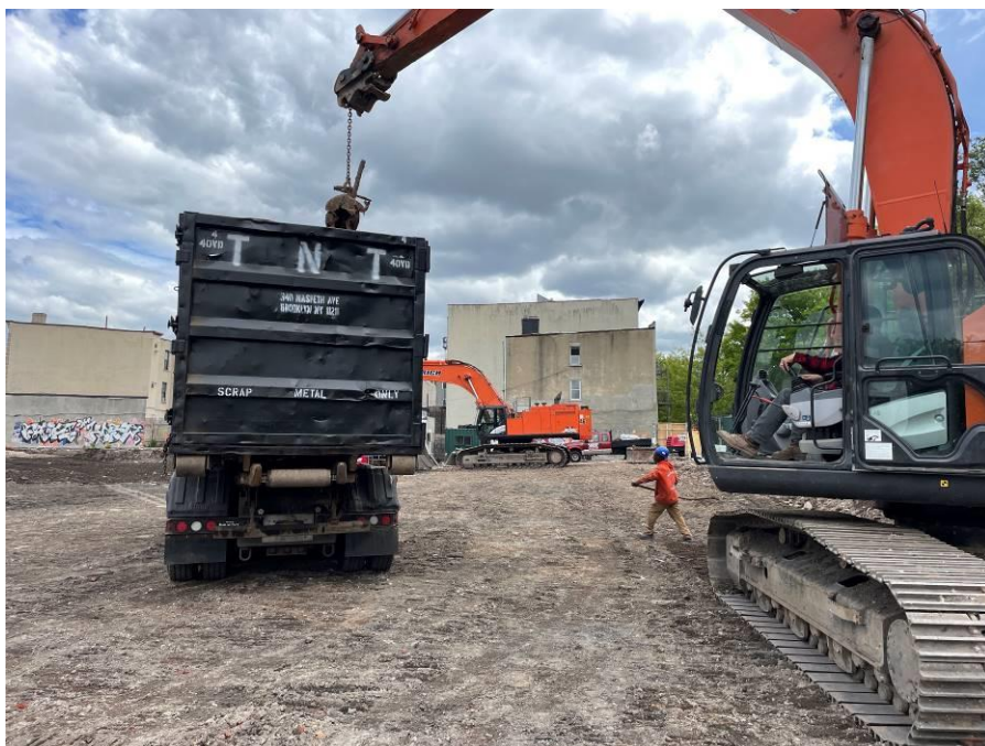
Photo 2: Mayrich exporting previously-decommissioned UST carcasses in the southern portion of BCP Site No. C224220 (facing east)
