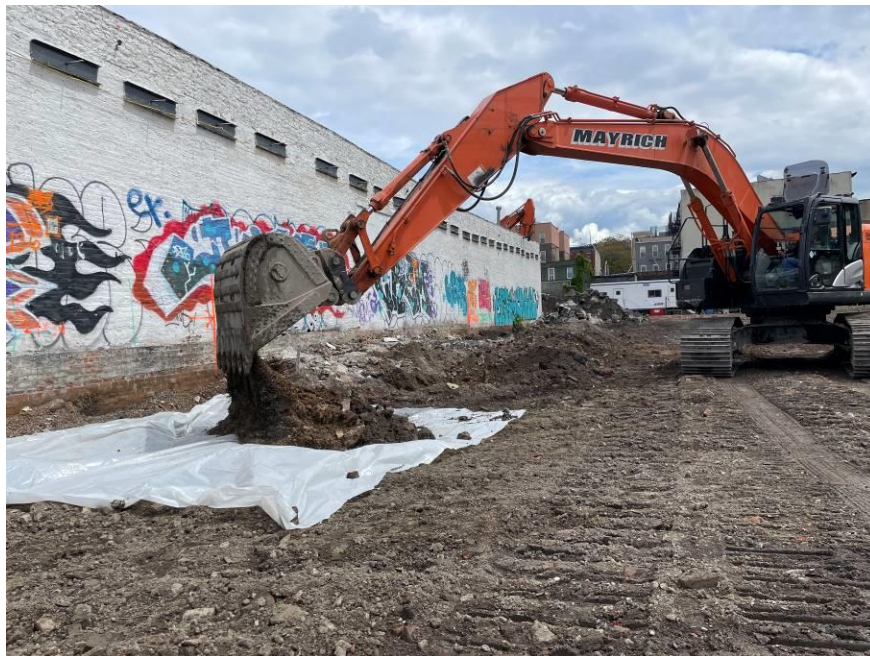
Photo 2: Mayrich performing remedial excavation in the northern portion of BCP Site No. C224220 (facing east)
