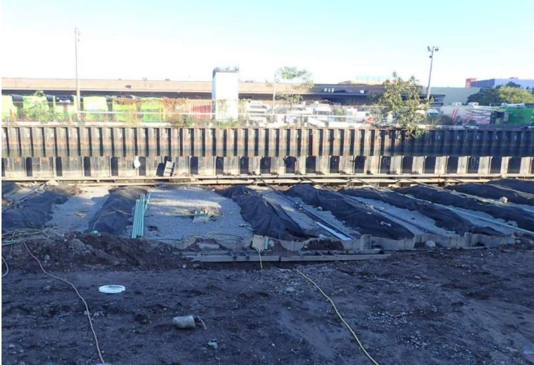
Photo 1: View of bulkhead installation progress near wale no. 5 (facing east).
