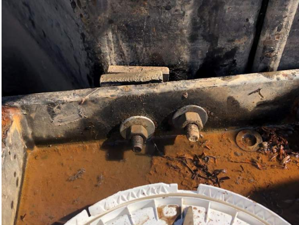
Photo 1: View of shim and washer installation (facing east).
