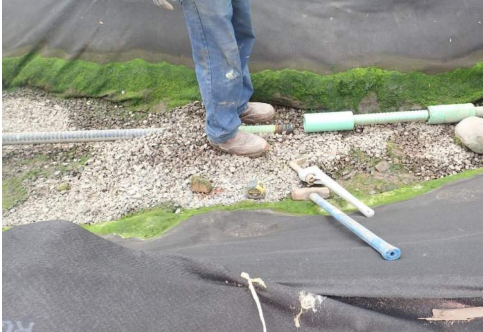
Photo 1: View of tie rod extension installation (facing south).
