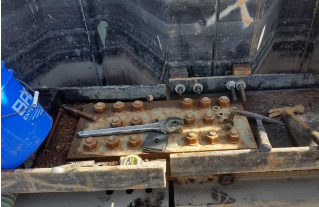
Photo 1: View of bolt, washer and shim installation (facing east).
