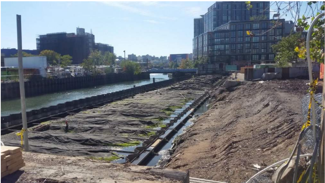
Photo 2: View of the bulkhead installation progress (facing south).
