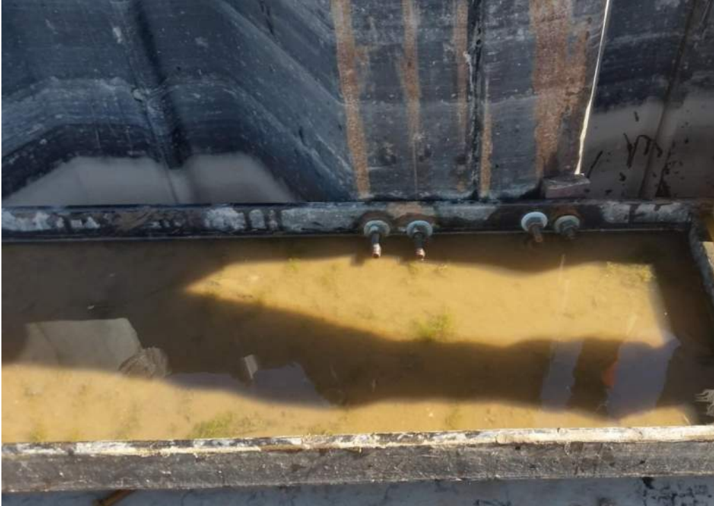
Photo 1: View of washer installation along bulkhead wale no. 2 (facing east).
