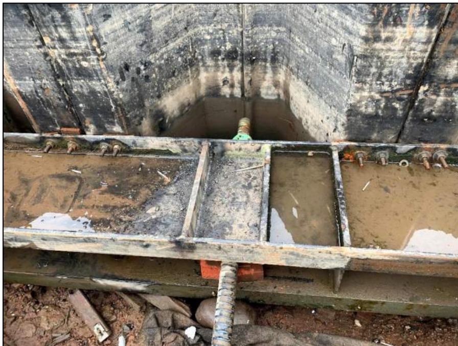
Photo 2: General view of bulkhead wale splice installation (facing east).
