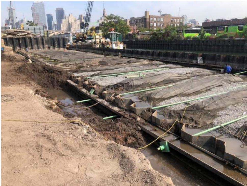
Photo 2: View of installed tie rods through wale no. 5 (facing northeast).
