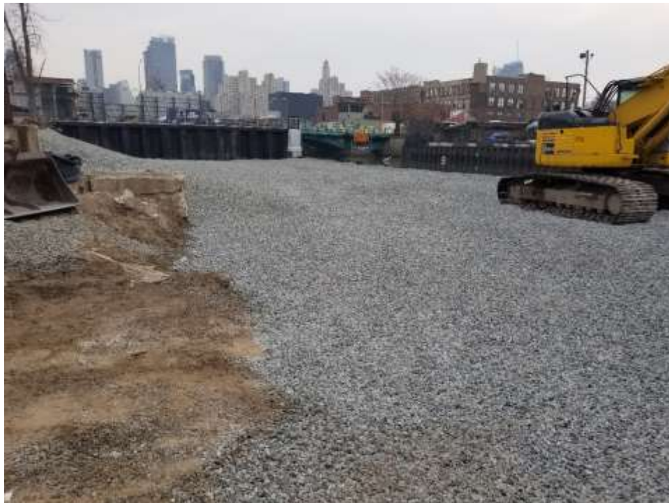
Photo 2: View of site (facing northeast).
