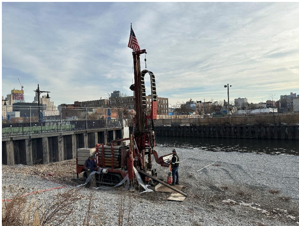
Photo 1: ADT advancing soil boring SSB-01 in the northeastern part of the site (facing northeast)
