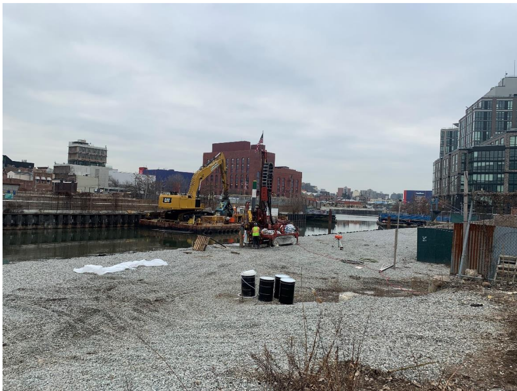
Photo 1: ADT installing down gradient monitoring well SMW-06DGS (facing southeast)
