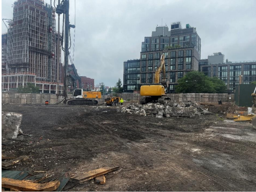
Photo 1: General view of C&D debris stockpile (facing south)
