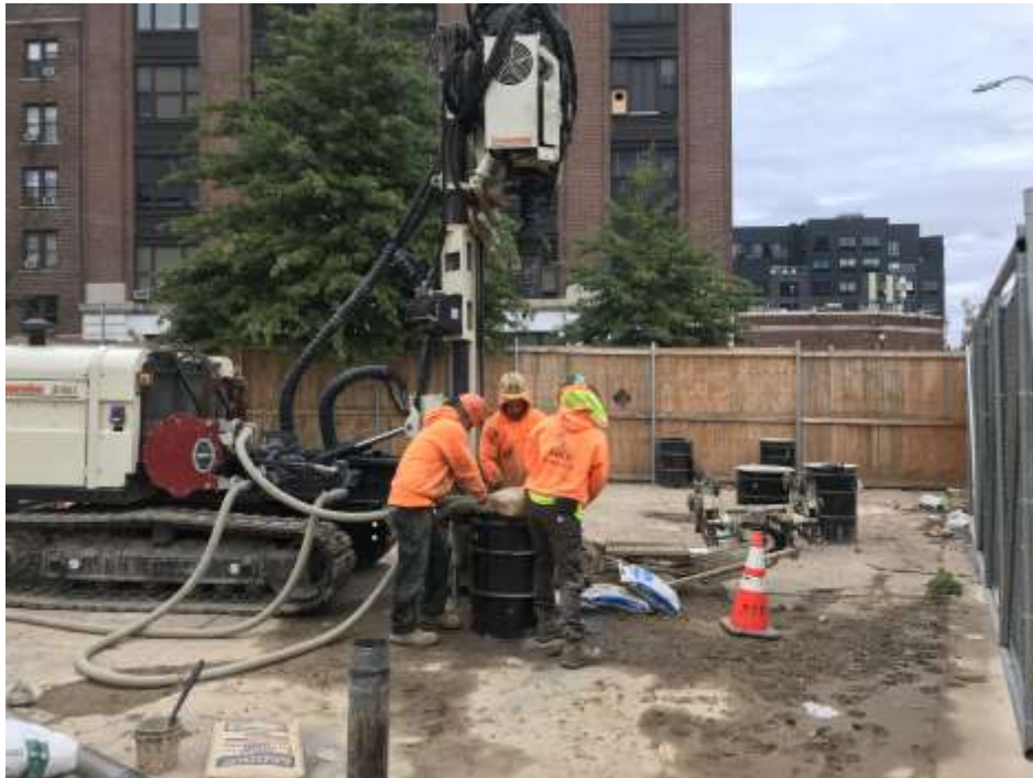
Photo 1: AARCO Installing injection well IP-02 (facing east).
