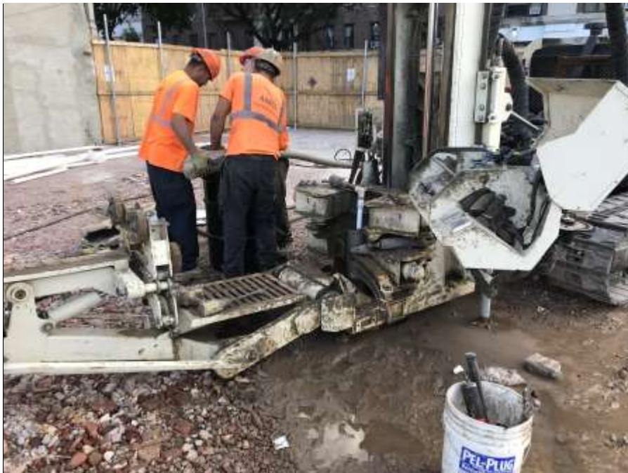
Photo 2: AARCO mixing grout prior to backfilling the annulus of MW-202 (facing northeast).
