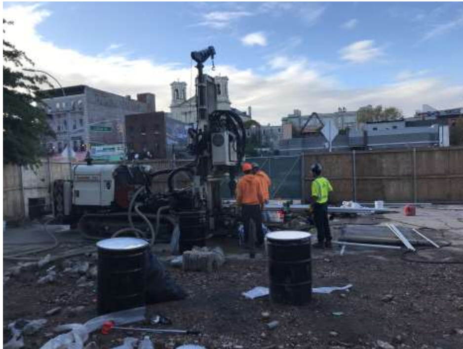
Photo 1: AARCO installing injection well IP-07 (facing south).
