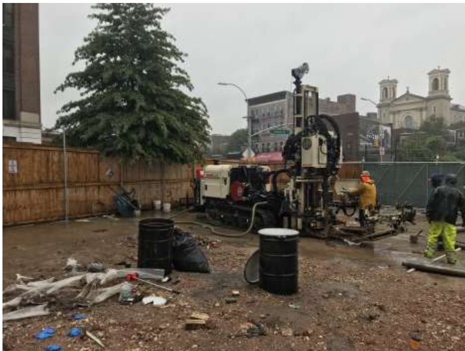
Photo 2: AARCO advancing boring IP-07 (facing southeast).
