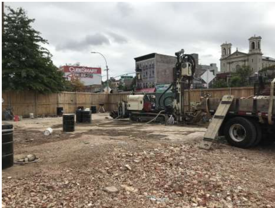
Photo 2: AARCO advancing boring IP-03 (facing east).
