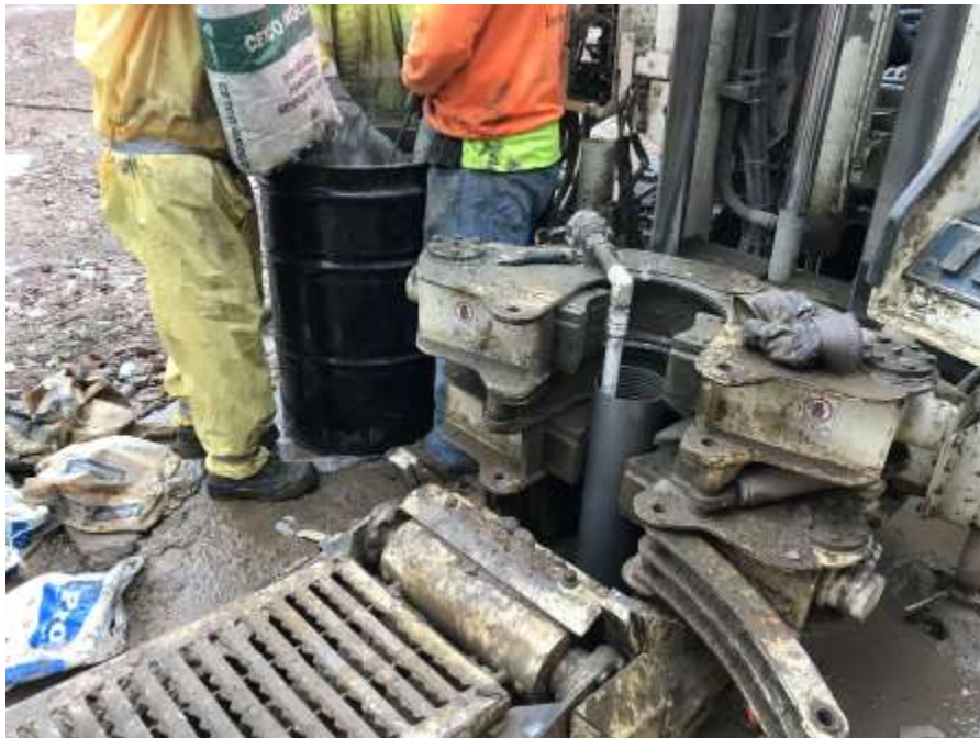
Photo 2: AARCO using a tremi pipe to backfill the annulus of IP-11 with a bentonite-grout slurry.
