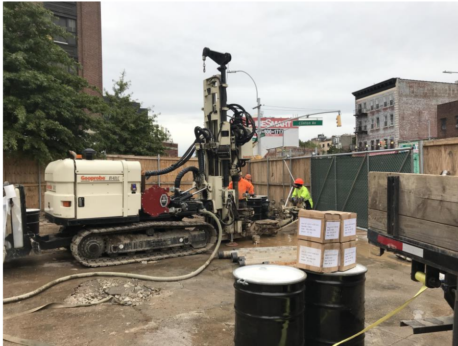
Photo 1: AARCO advancing IP-02 (facing east).
