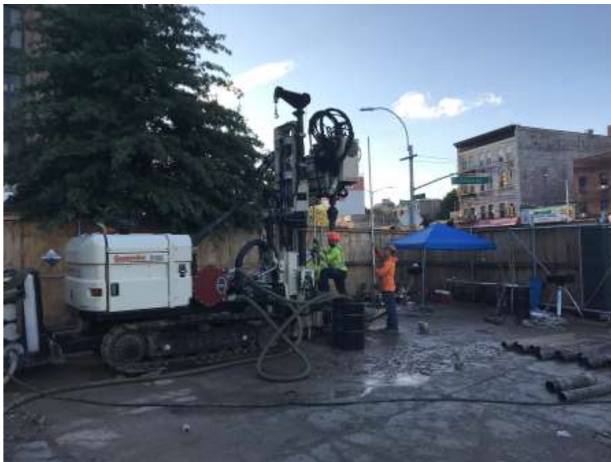
Photo 2: AARCO installing injection well IP-06 (facing southeast).
