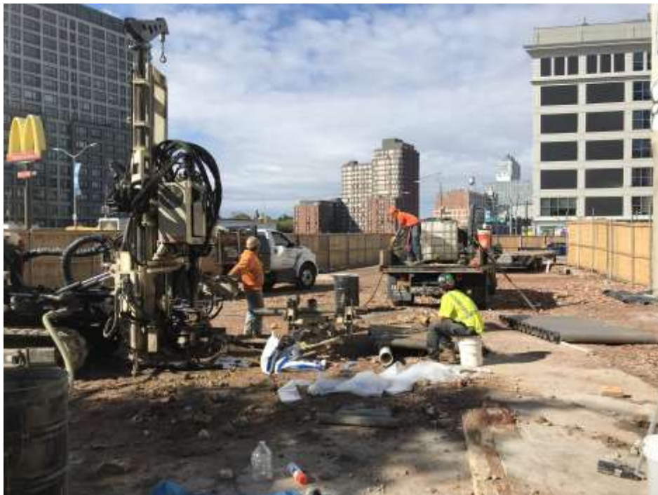
Photo 2: AARCO advancing IP-12 (facing west).
