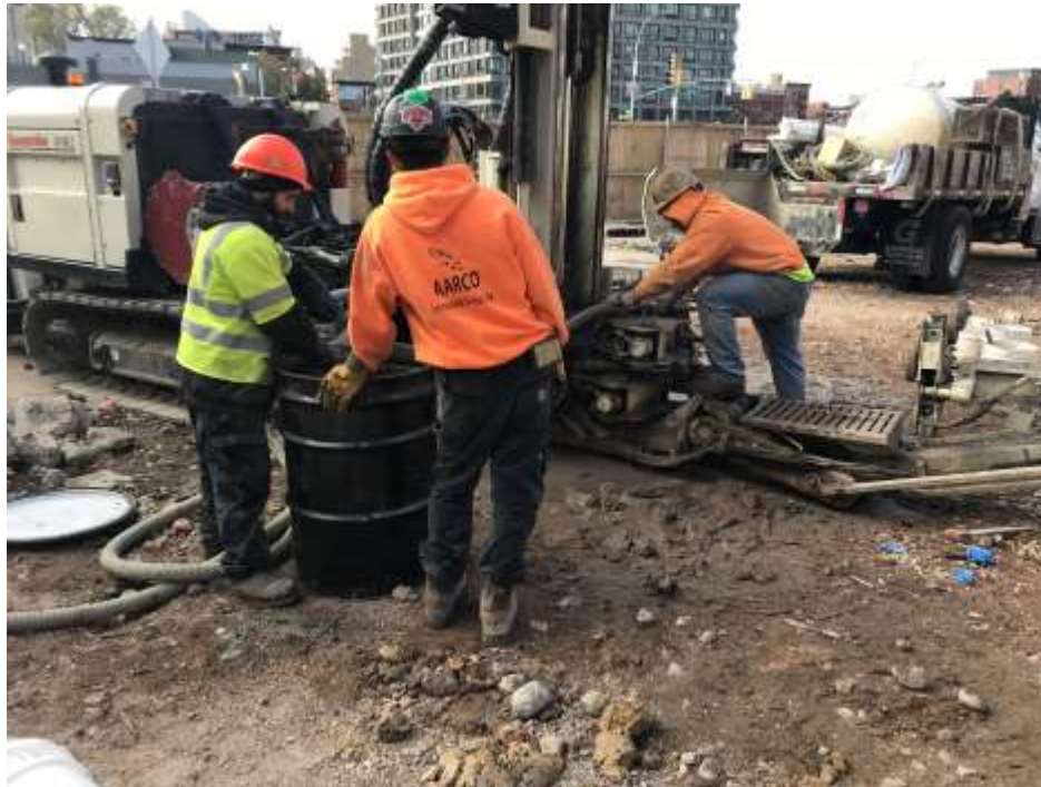
Photo 1: AARCO installing injection well IP-12 (facing south).
