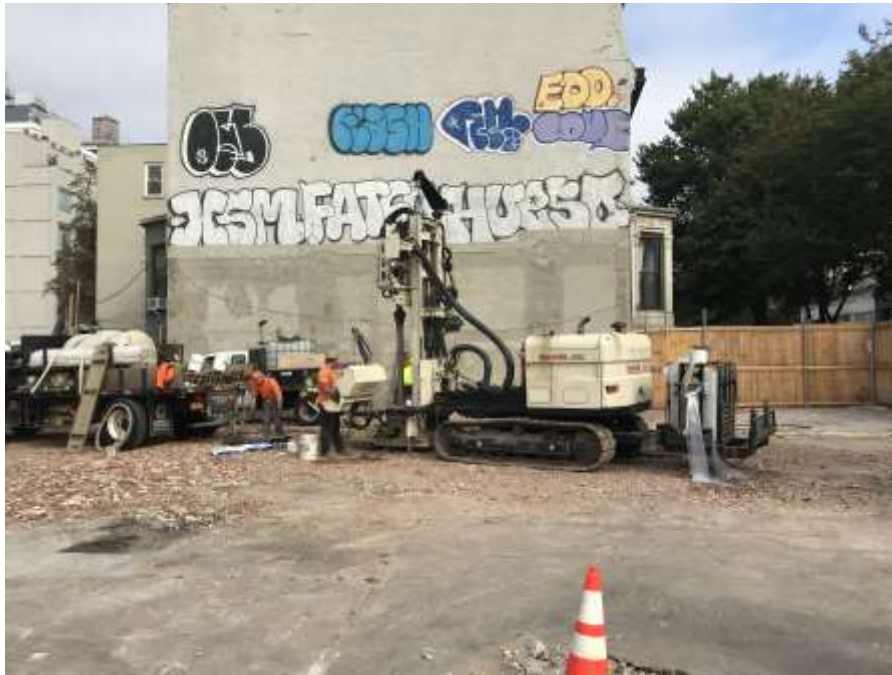
Photo 1: AARCO drilling MW-202 (facing north).
