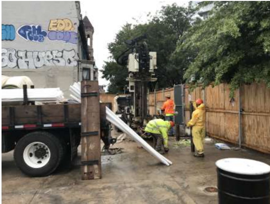
Photo 1: Advancement of injection point IP-11 (facing north).
