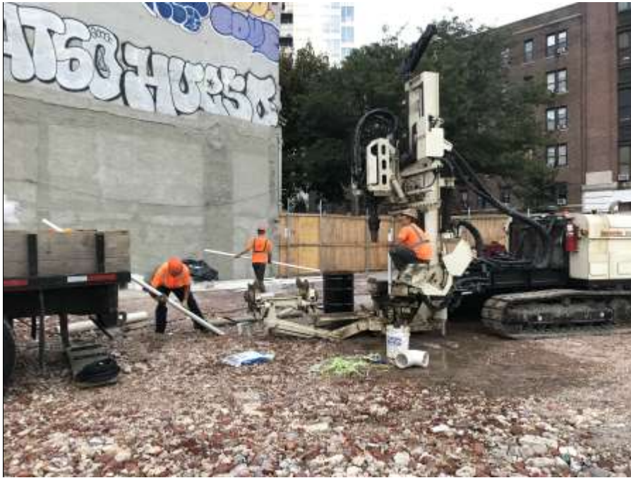
Photo 1: AARCO installing monitoring well MW202 (facing northeast).
