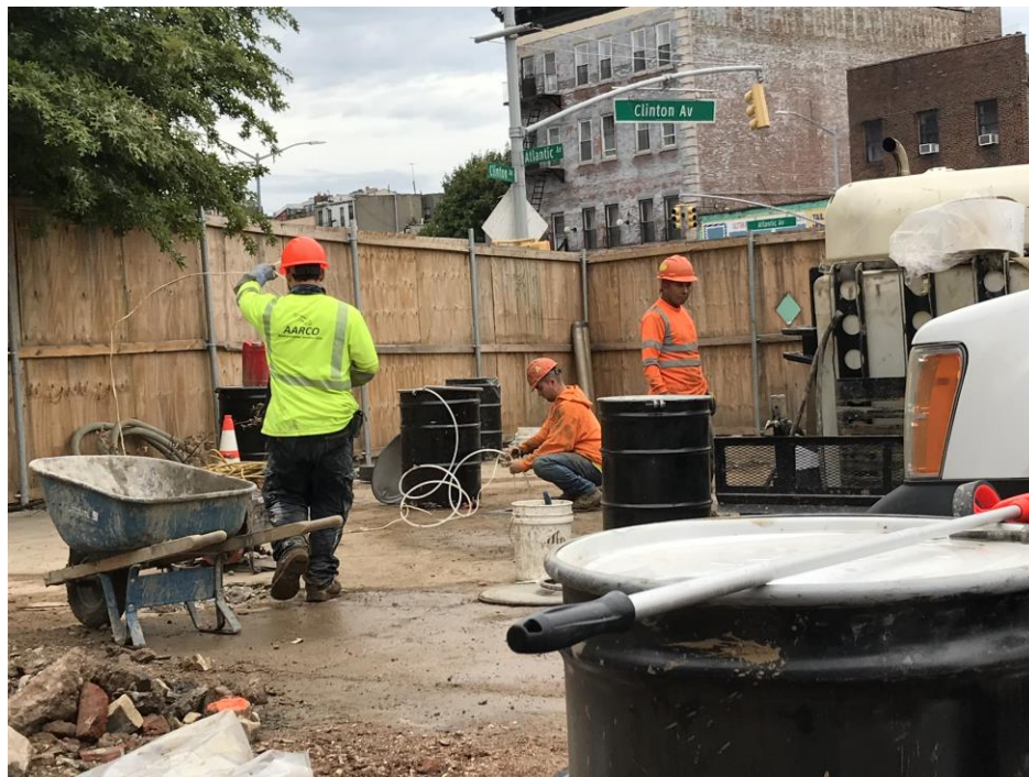
Photo 2: AARCO developing injection point IP-06 (facing southeast).
