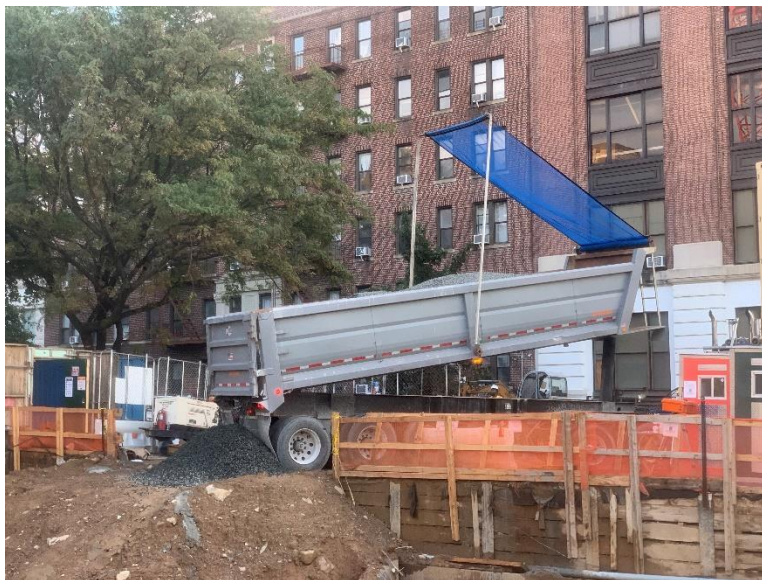
Photo 44: Import of 3/4-inch quarry stone (facing northeast). Taken on 09/11/2020.
