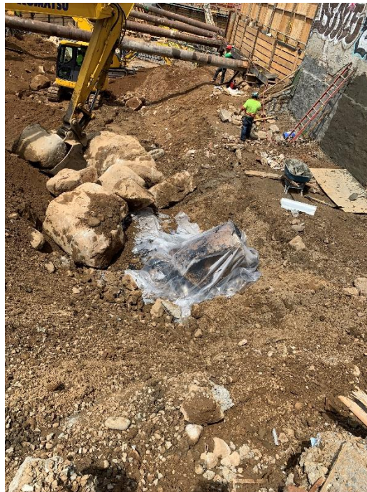
Photo 30: View of the encountered 550-gallon UST covered with polyethylene sheeting located in the northeastern part of the site. Taken on 06/04/2020.
