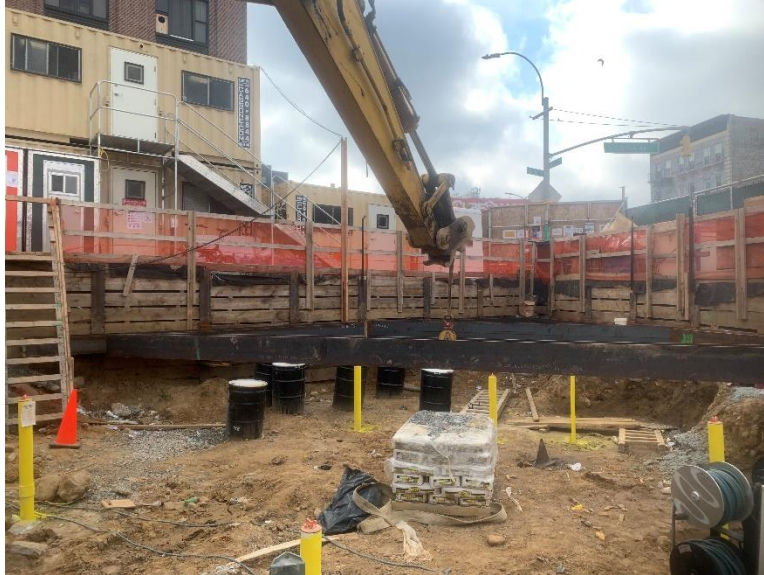
Photo 39: General view of installed groundwater monitoring wells and SVE wells (facing southeast). Taken on 08/11/2020.
