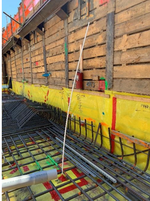
Photo 33: View of vapor monitoring point (VMP) installation in the western part of the site. Taken on 06/12/2020.
