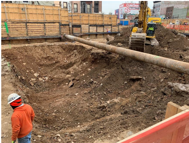
Photo 24: Excavation of non-hazardous fill from grids WC02 and WC03 for future off-site disposal (facing southeast). Taken on 04/23/2020.
