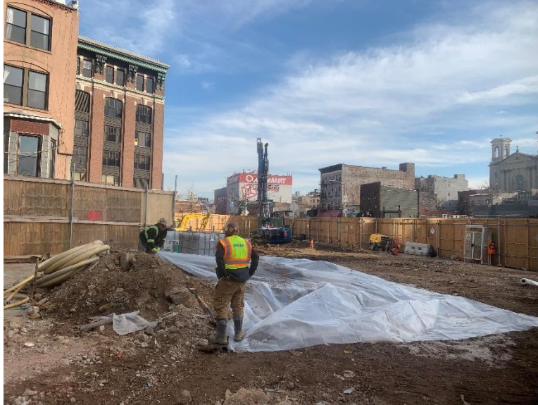
Photo 9: Kingdom preparing stockpile for soil generated during air rotary drilling (facing east). Taken on 01/24/2020.
