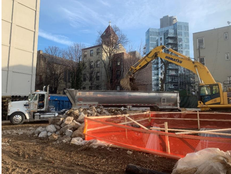
Photo 13: Off-loading of hazardous lead-impacted historic fill material from WPSB-01 and SB-107A (facing northeast). Taken on 02/12/2020.
