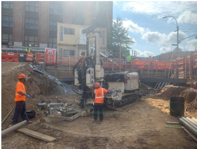
Photo 38: Photo 2: AARCO advancing soil vapor extraction (SVE) well SVE-5 (facing southeast). Taken on 07/15/2020.
