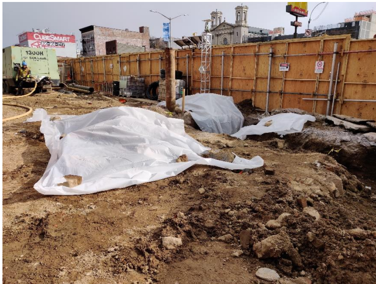
Photo 16: Stockpiles of non-hazardous historic fill material covered with poly sheeting in southwestern corner of the site (facing southeast). Taken on 02/29/2020.
