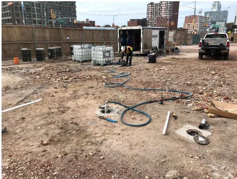
Photo 4: Regenesis injecting Nutrisulfate at injection point IP-13 (facing southwest). Taken on 11/07/2019.
