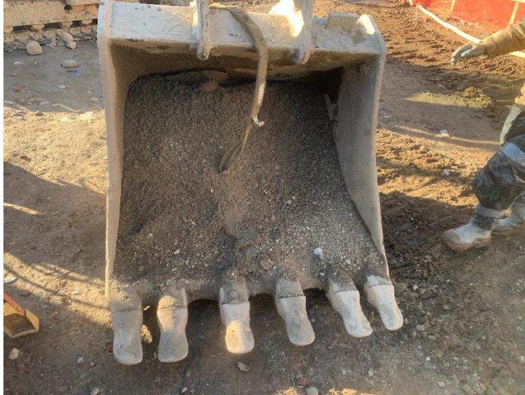
Photo 15: Collected air rotary drilling spoils prior to stockpiling (facing west). Taken on 02/27/2020.
