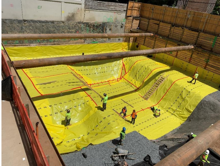
Photo 29: Installation of the vapor barrier in the northern part of the site (facing north). Taken on 05/21/2020.
