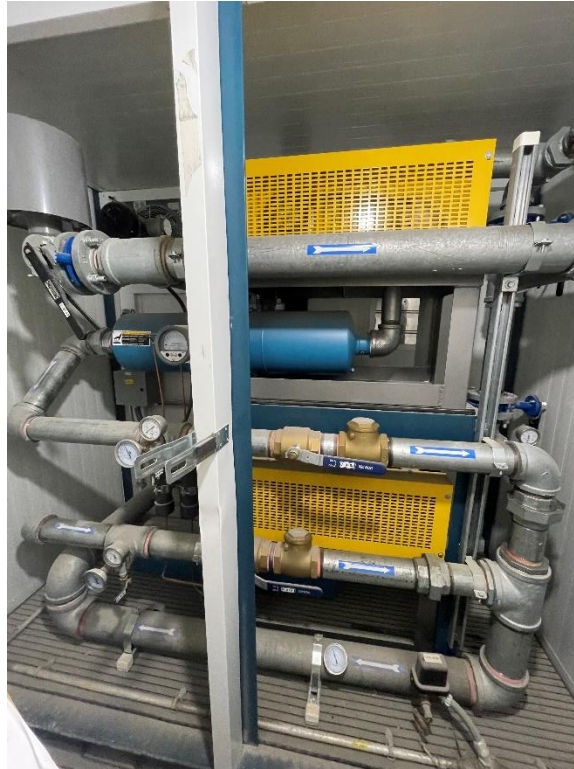
Photo 55: General view of blowers for the SVE system (facing south). Taken on 11/22/2021.
