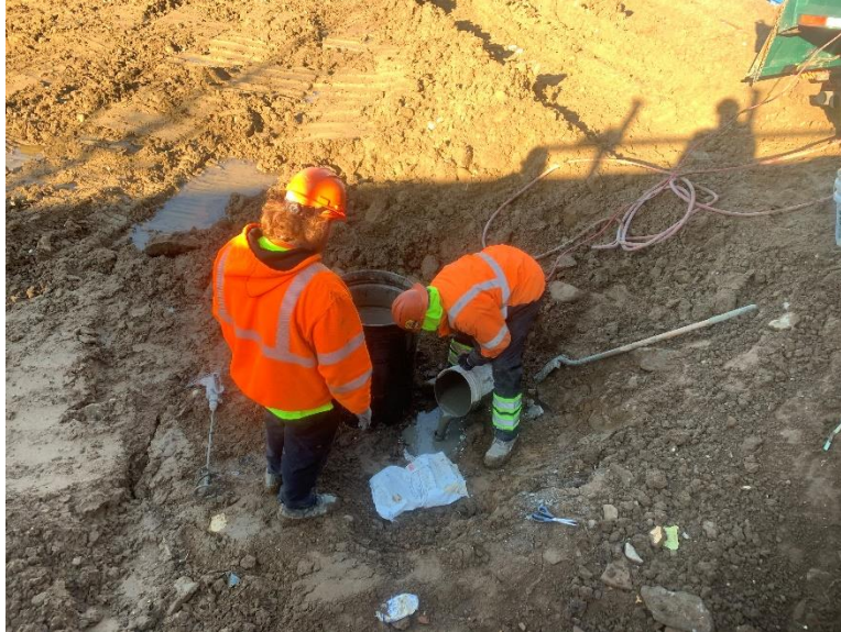
Photo 17: Decommissioning of injection point (IP-11) in the southeastern section of the site (facing west). Taken on 03/04/2020.
