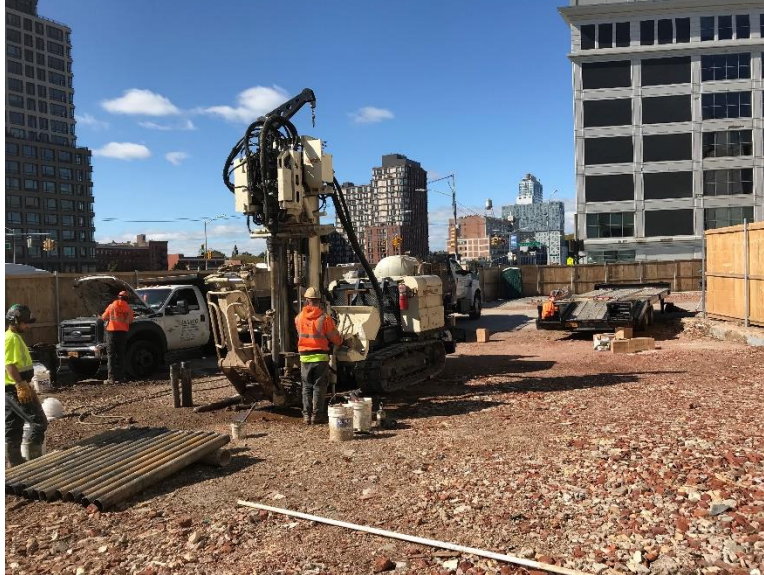
Photo 3: AARCO advancing groundwater injection point IP-10 (facing west). Taken on 10/18/2019.
