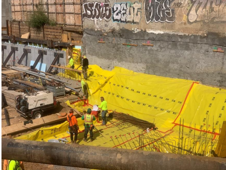
Photo 45: Vapor barrier installation in the eastern section of the site (facing northwest). Taken on 09/21/2020.
