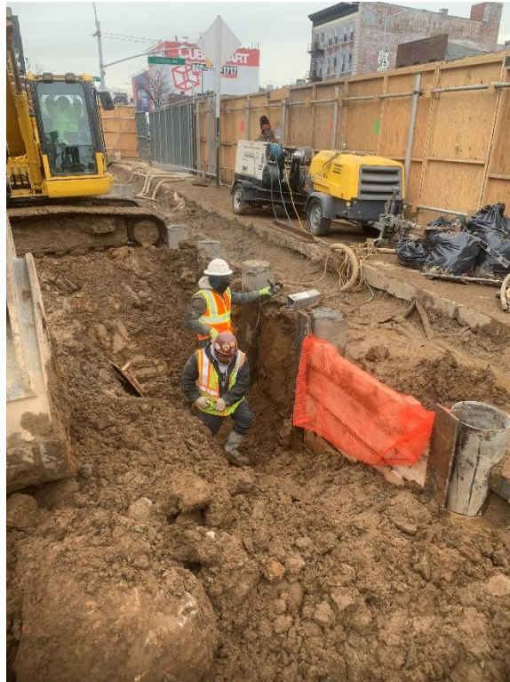
Photo 12: Excavation of non-hazardous historic fill material for the installation of lagging (facing southeast). Taken on 02/05/2020.
