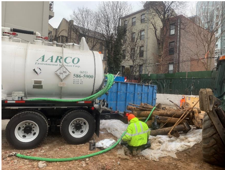
Photo 10: AARCO cleaning and disposing of hydraulic pistons encountered during mass excavation (facing northeast). Taken on 01/31/2020.
