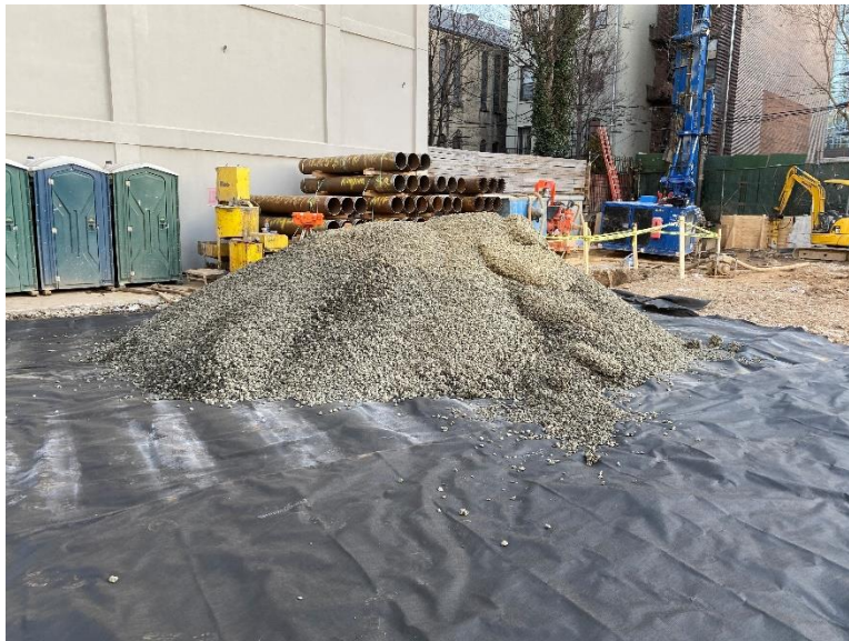
Photo 14: Imported \frac{3}{4} -inch quarry stone to be used for the site entrance track pad (facing north). Taken on 02/20/2020.
