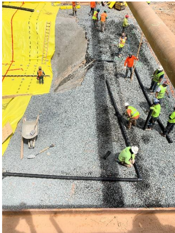
Photo 28: Installation of four-inch sub-membrane depressurization system (SMDS) piping on top of a six-inch-thick stone subgrade and geotextile fabric in the northwestern part of the site (facing east). Taken on 05/22/2020.
