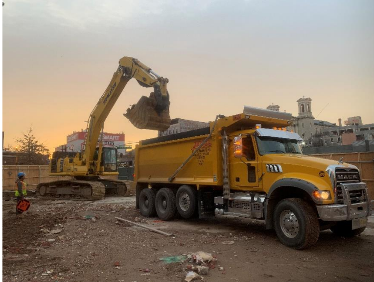
Photo 7: Off-loading of non-hazardous historic fill material from grid WC-05 (facing southeast). Taken on 01/07/2020.
