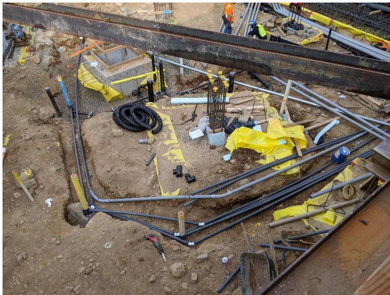
Photo 46: SVE well and piping installation in the southeastern section of the site (facing west). Taken on 09/25/2020.
