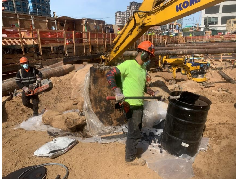
Photo 35: Cleaning of USTs identified during excavation prior to off-site disposal (facing north). Taken on 06/15/2020.
