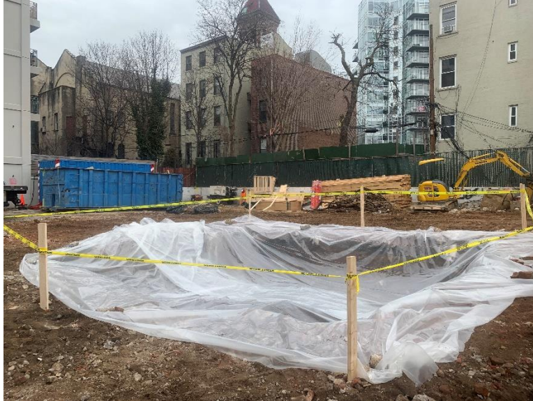
Photo 11: Excavation of hazardous lead-impacted hot spot, SB-107A, taped off and covered with poly-sheeting (facing northeast). Taken on 02/04/2020.
