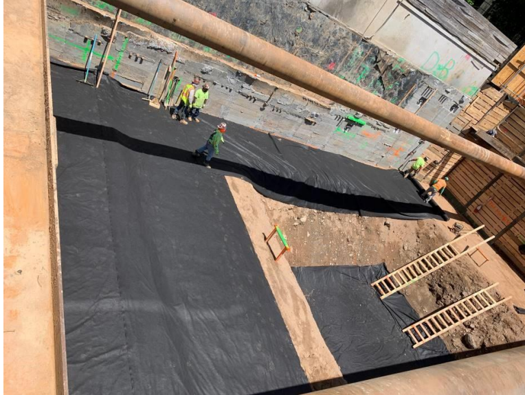
Photo 27: Installation of geotextile fabric prior to quarry stone placement in the northwestern section of the site (facing northeast). Taken on 05/21/2020.
