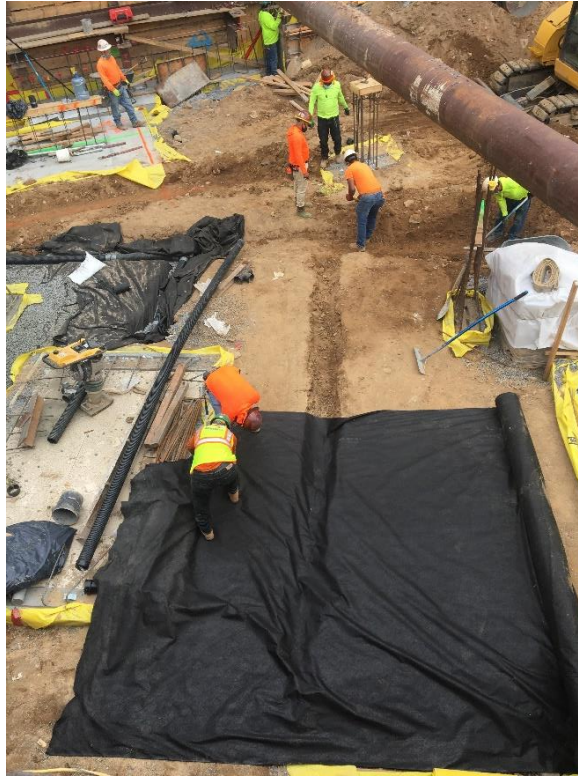
Photo 41: Excavation of SMDS piping and placement of geotextile fabric in the central part of the site (facing north). Taken on 08/31/2020.
