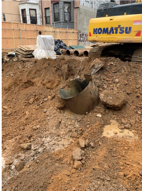
Photo 21: View of the encountered 550-gallon underground storage tank (UST) located in the southeastern part of the site. Taken on 03/20/2020.
