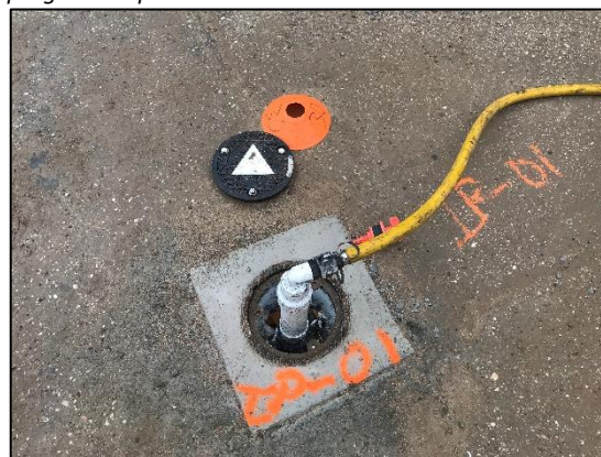
Photo 4: Closeup on a typical Injection Well. White PVC attachments were used to hook up injection hoses to the wells.
