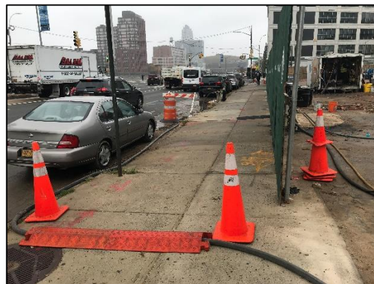
Photo 6: Water source (hydrant) on Atlantic Avenue being fed to injection trailer.
