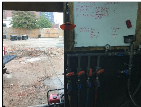
Photo 2: Another overview of the worksite, but this time from inside the injection trailer. Also, flow meters (under orange valves) were used inside the trailer to monitor progress on points.
