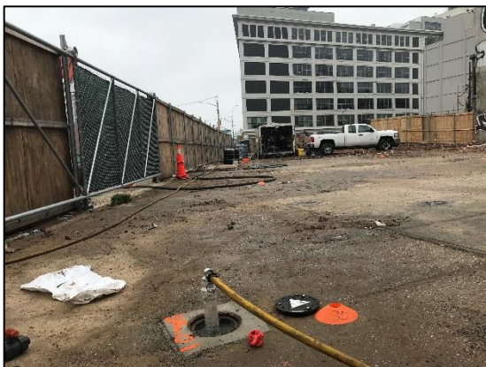
Photo 1: Overview of worksite, and IP-1 being pumped on. Orange circular cones were used to mark Injection Wells.
