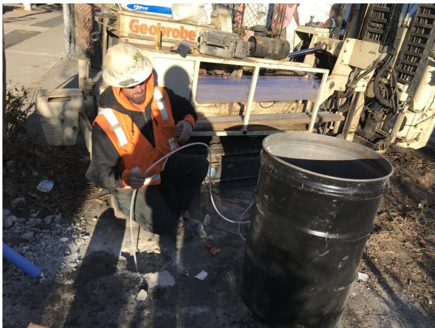
Photo 8, 11/21/2017: AARCO developing groundwater monitoring well 16MW3, facing northwest.
