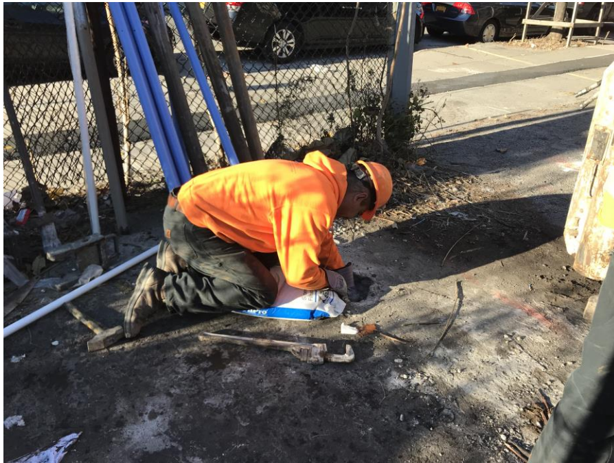
Photo 7, 11/21/2017: AARCO installing groundwater monitoring well 16MW3, facing west.
