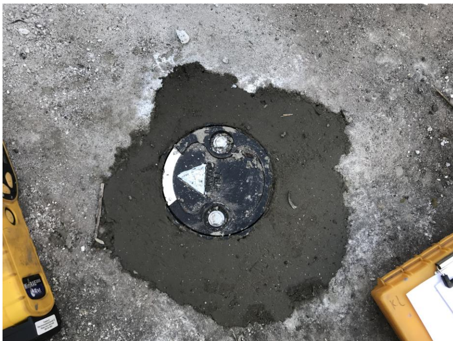
Photo 14, 3/12/2017: Finished manhole cover for monitoring well 16MW3.
