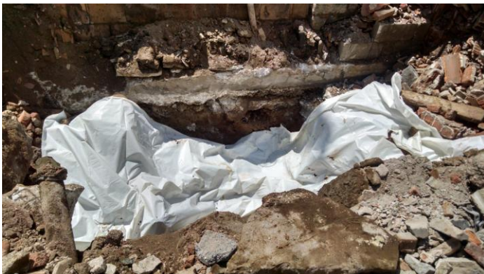
Photo 17: Plastic in excavation before backfill in case further excavation is required based on lab
