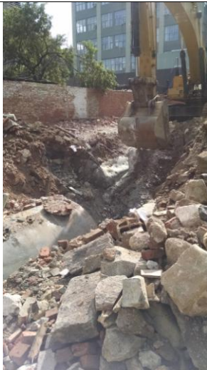
Photo 1: Excavation of Tank 1/Tank 2 in foreground
