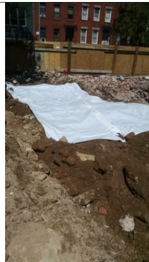
Photo 16: Plastic for cont. soil removal
