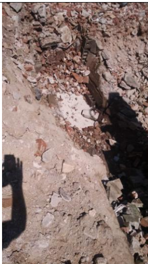
Photo 15: Speedy Dry to soak oil prior to further excavation
