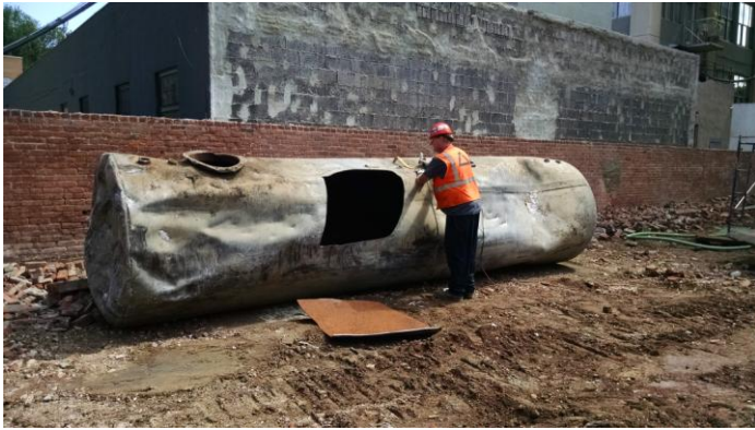
Photo 7: Tank 1 Cleaning
