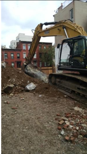
Photo 3: Removal of Tank 1
