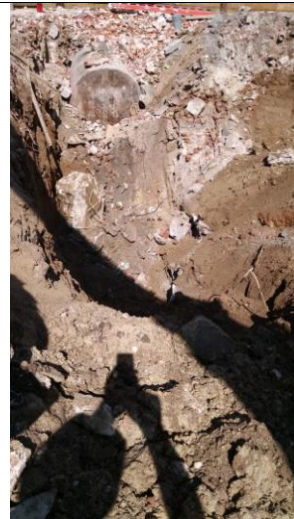
Photo 8: Tank 2 Shared E/W Sidewall with Tank 1
