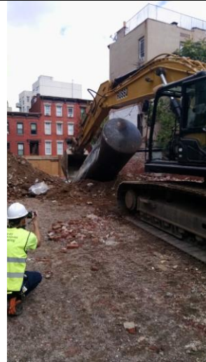
Photo 4: Removal of Tank 1
