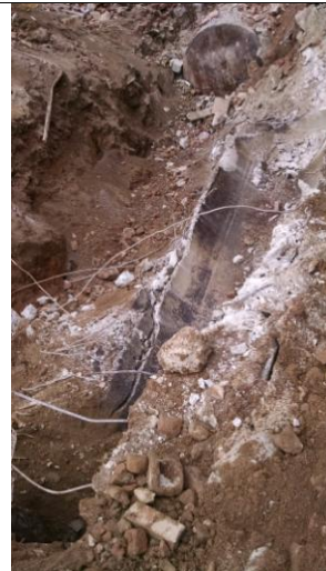
Photo 6: Tank 1 Post Excavation
