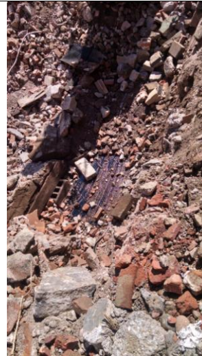
Photo14: Vault Slab and block sidewalls
