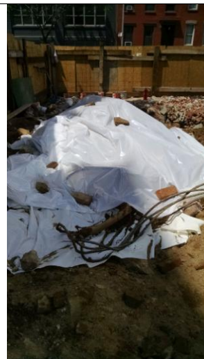
Photo 18: Cont. Soil pile pending disposal
