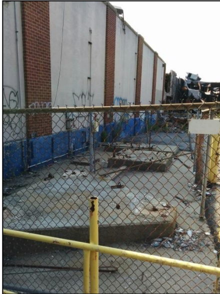
Photograph 5: Concrete pads at former liquid nitrogen tank locations on the eastern portion of the Site, facing south.
