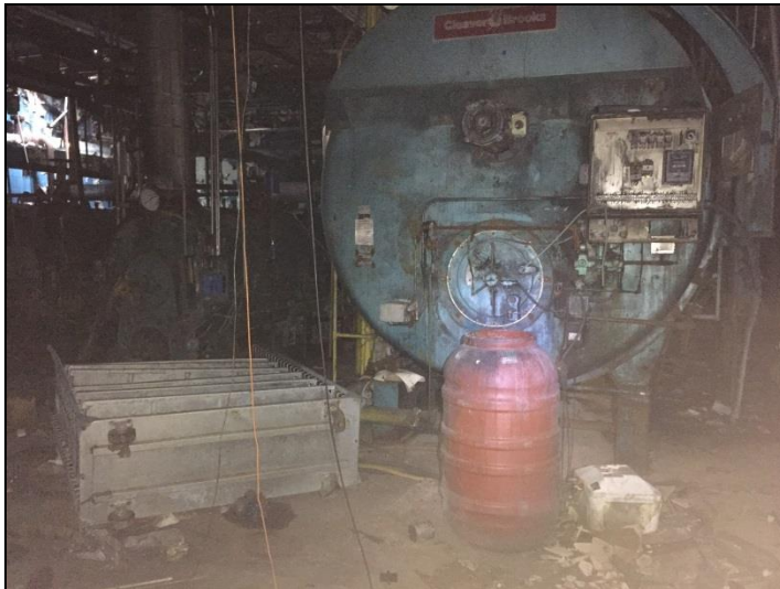
Photograph 7: Former boiler room in the northwestern portion of the Site buildings.
