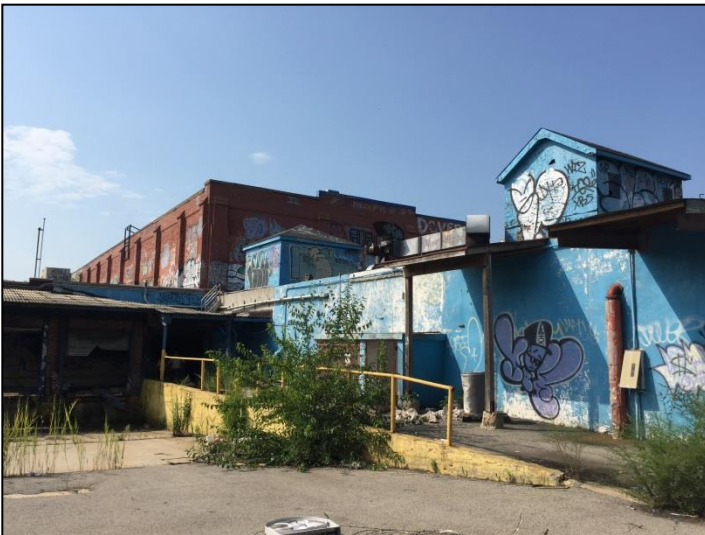
Photograph 3: Former receiving area on the western portion of the Site, facing southwest.
