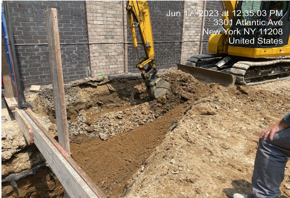
3 - Backfilling following completion of excavation.
