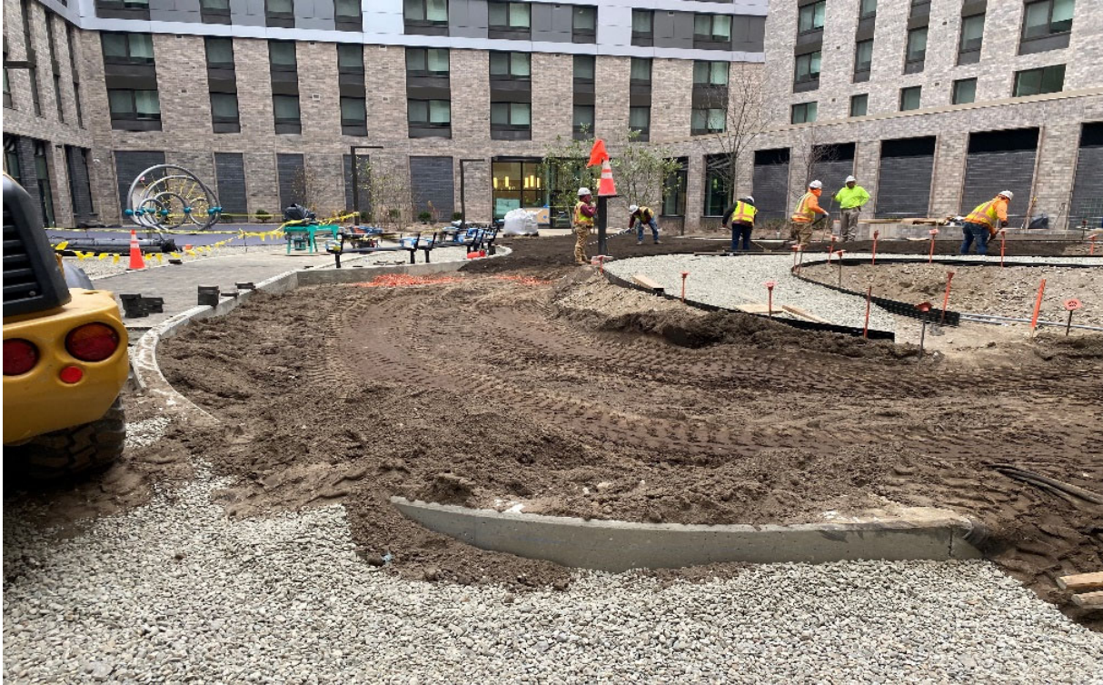
7 - Formwork for courtyard sidewalks, view facing northwest.
