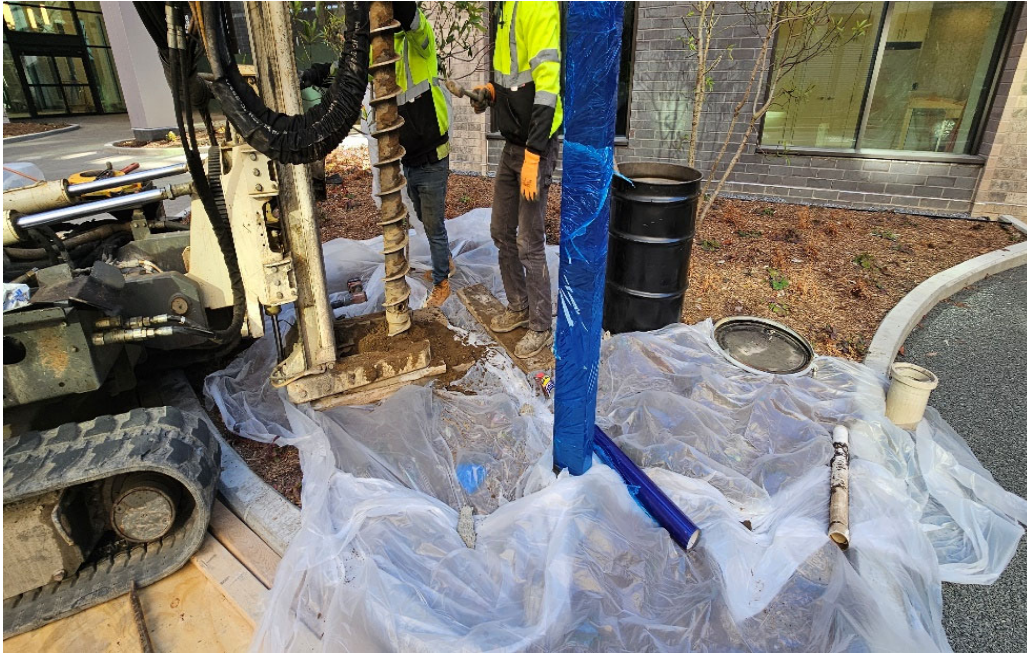
11 - Redrilling a groundwater monitoring well.
