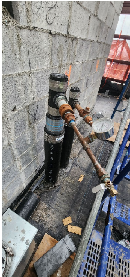
15 – SSDS and SVE riser pipe pressure testing.
