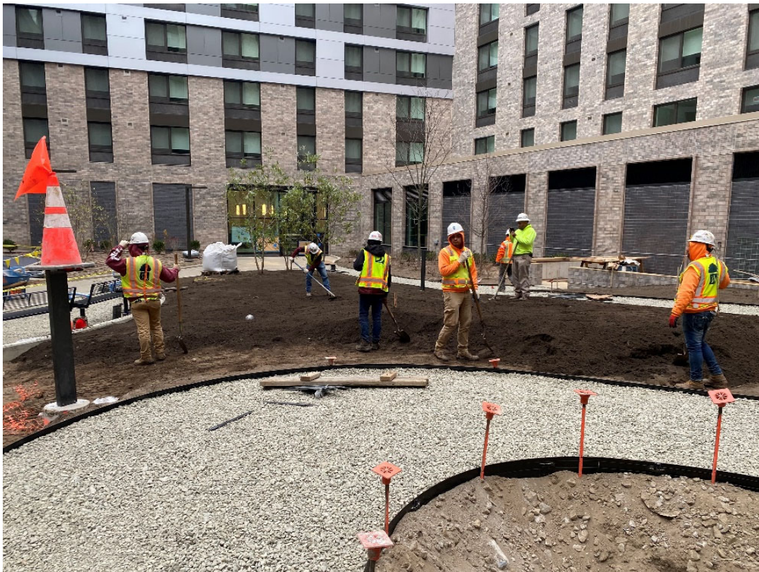
8 - Placing imported topsoil over imported clean fill, view facing northwest.
