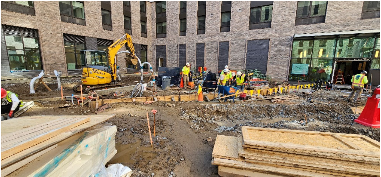
6 - Formwork for courtyard sidewalks, view facing southwest.
