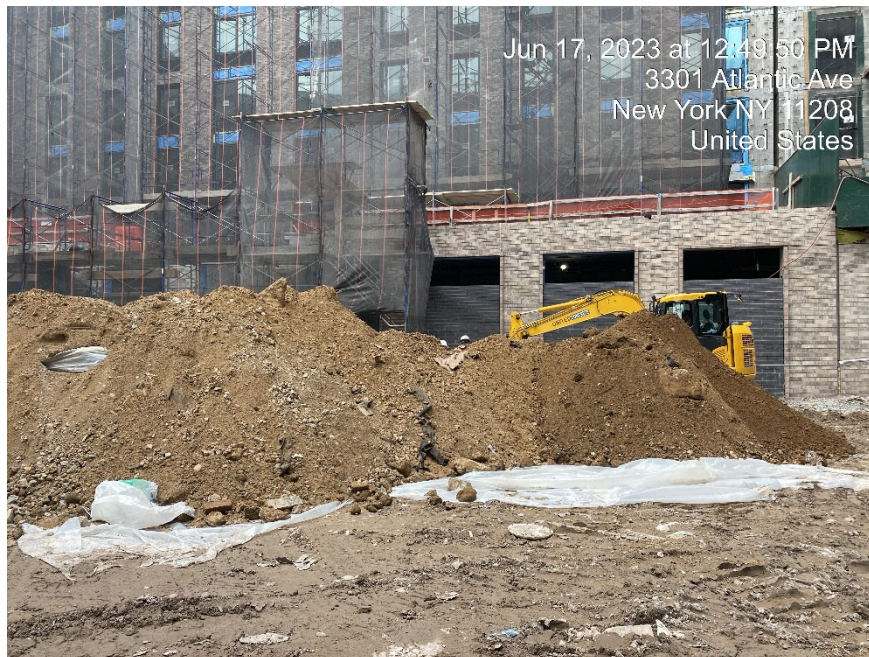
2 - Temporary stockpile of clean fill on polyethylene sheeting prior to use as backfill following completion of excavation.
