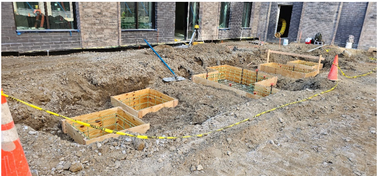
4 – Formwork for foundation elements, view facing southwest.
