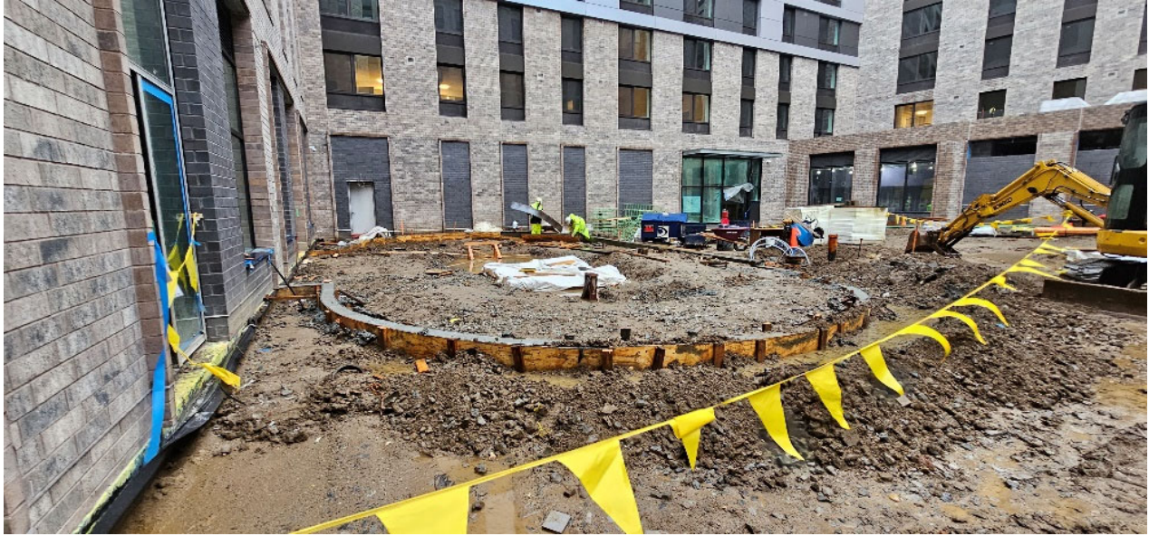
5 - Formwork for courtyard playground elements, view facing northwest.
