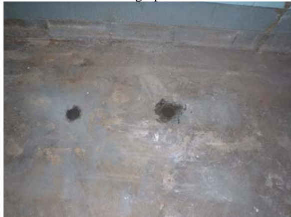
Basement slab restored
