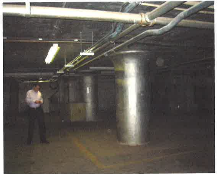
BASEMENT OF LARGE BUILDING
