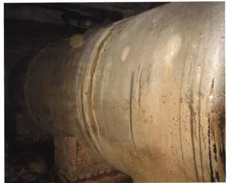
HEATING OIL TANK IN BASEMENT
