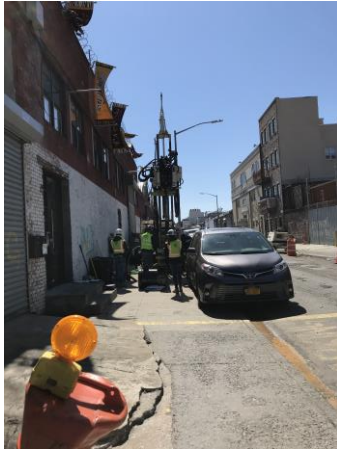
Photo 1: View of well installation at MW07.
