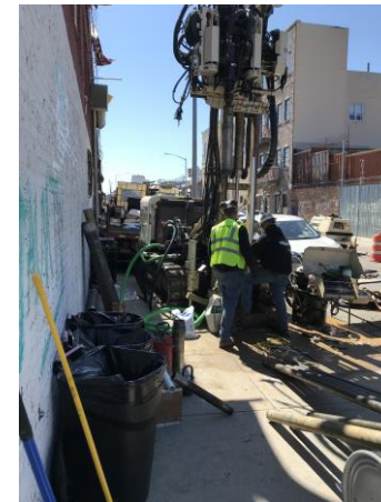
Photo 4: View of setting MW07.
