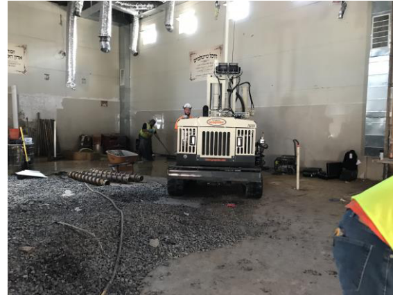
Photo 2: View of mobilization of Geoprobe 7822DT.
