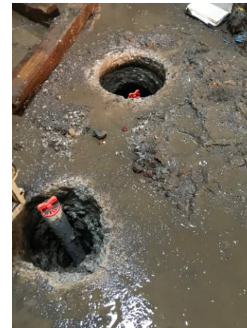
Photo 4: View of setting MW-05(S) and MW-05(I).
