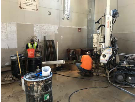
Photo 1: View of attempted installation of MW-01(I).
