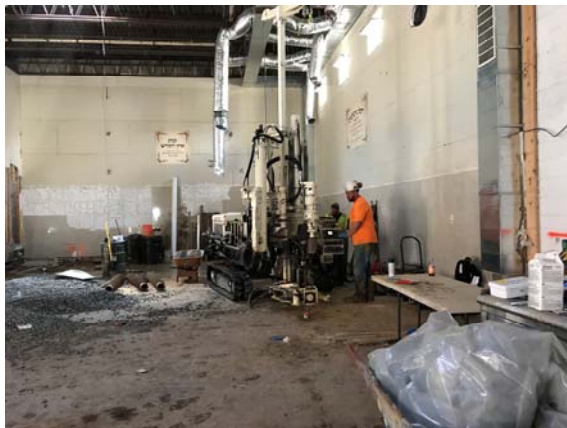
Photo 3: View of installation of MW-02(S).
