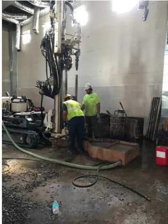
Photo 1: View of MW-02(D) installation.
