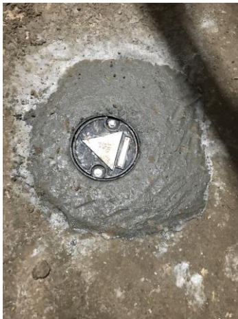
Photo 3: View of manhole cover installation.
