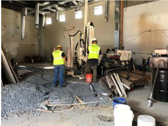
Photo 1: View of Geoprobe 7822DT mobilization to B04.
