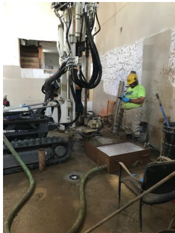
Photo 3: Attempted installation of MW-01(I).
