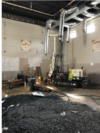
Photo 1: View of Geoprobe 7822DT mobilization to MW-01.
