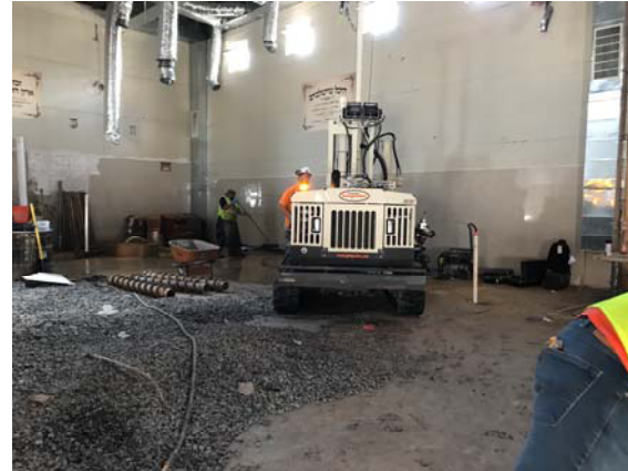
Photo 2: View of mobilization of Geoprobe 7822DT to MW-02.
