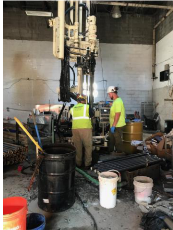
Photo 1: View of Geoprobe 7822DT mobilization to MW-05.
