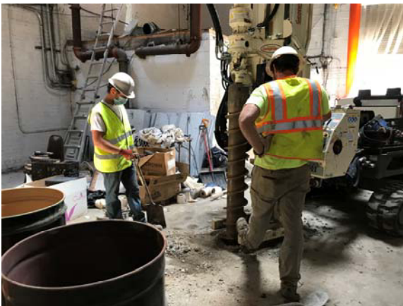
Photo 3: View of refusal encountered at MW05.
