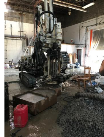
Photo 2: Alternate view of mud rotary setup.
