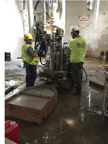
Photo 2: Alternate view of MW-02(D) installation.
