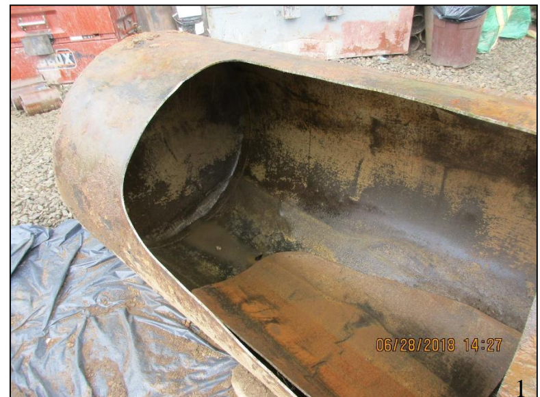
Photograph 4: Cut and cleaned tank prior to off-site disposal.
