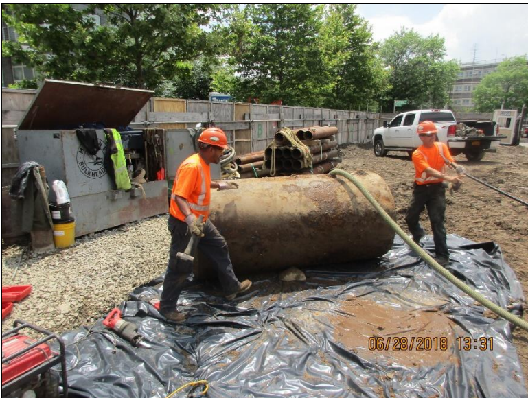
Photograph 3: Cleaning tank interior and exterior prior to off-site disposal.
