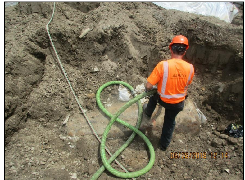
Photograph 2: AARCO Environmental Services pumping tank contents prior to removal.
