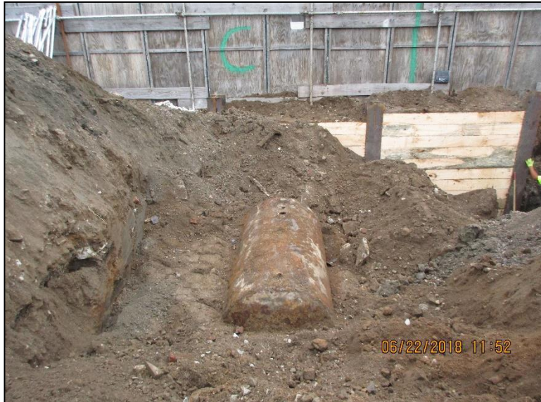
Photograph 1: 550-gallon underground storage tank encountered during excavation on the southern portion of the Site, facing south.
