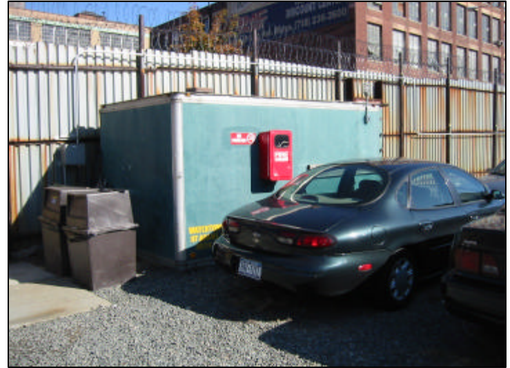
Photograph 2: Waiting area shelter.
