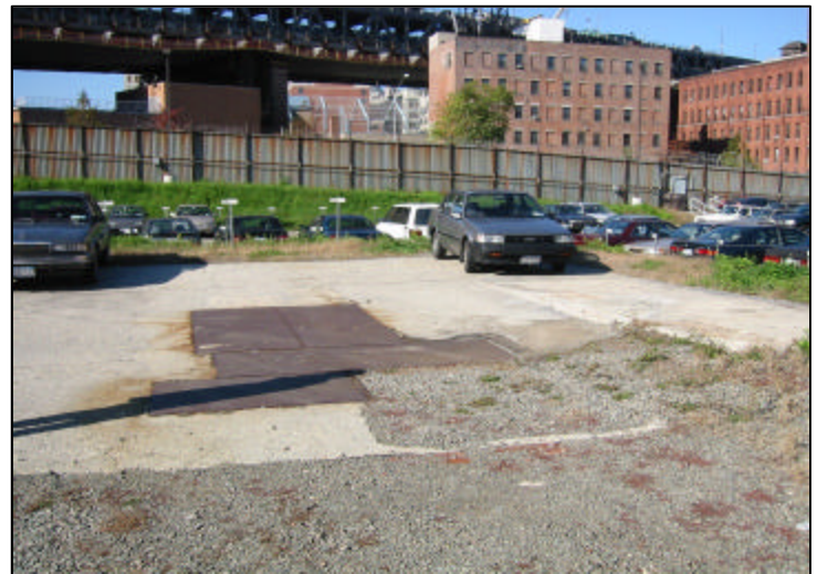
Photograph 4: Four steel plates on the concrete pad.
