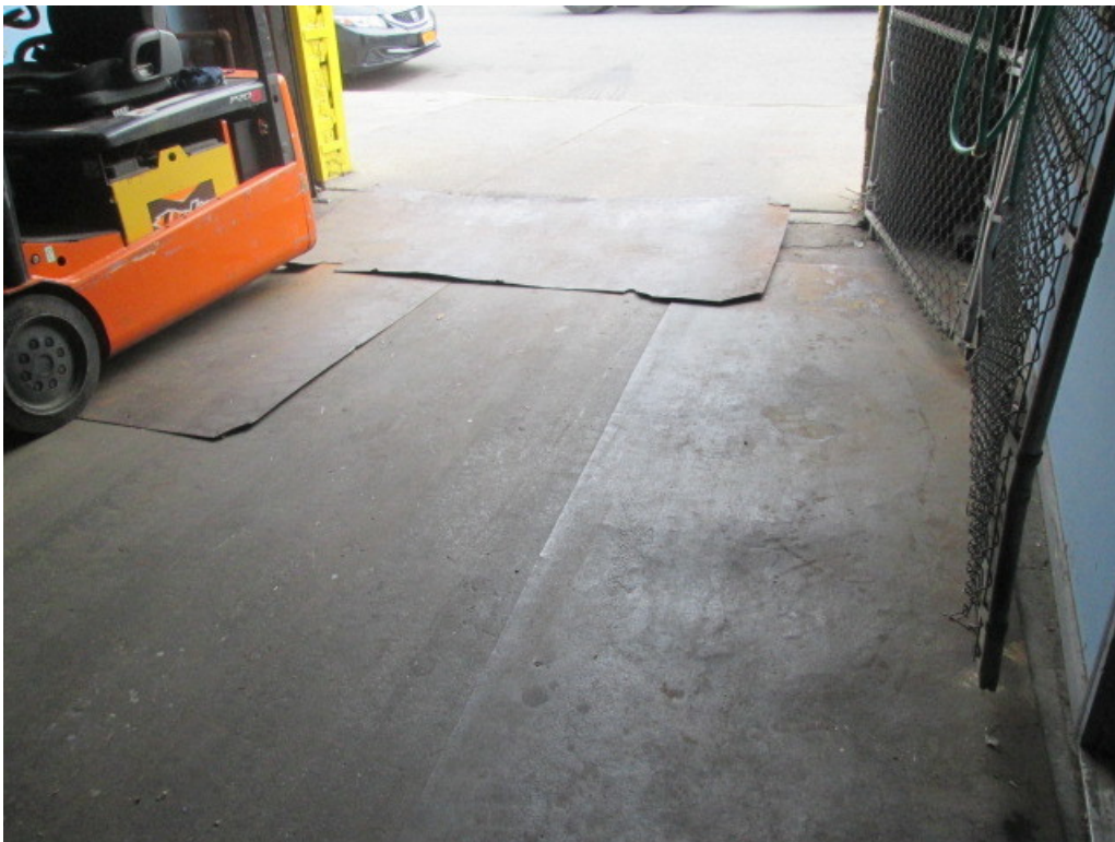
Steel plates covering front area of warehouse for support
