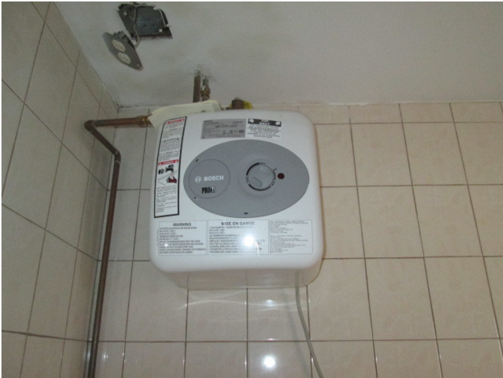
Electric hot water heater
