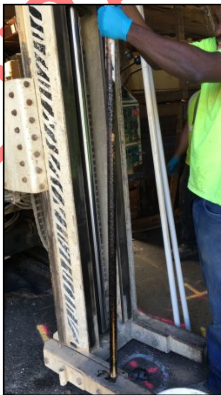
8 : Temp. well installed in MW-8 with fuel oil on PVC
