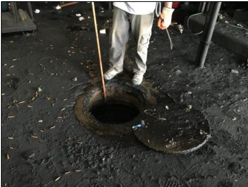
13 : Catch basin opened
